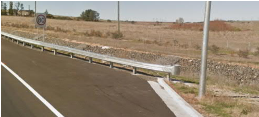
Figure 4-13 Existing safety barrier
