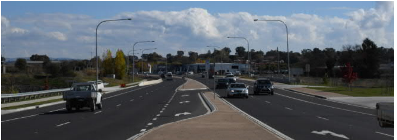
Figure 4-1 Recently completed highway upgrade at Kelso
