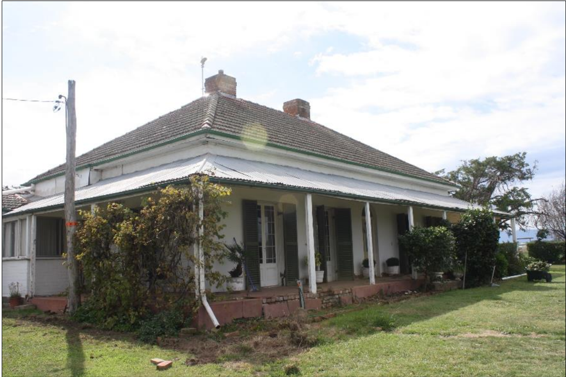
Figure 4-4: Violet Hill, facing north east
