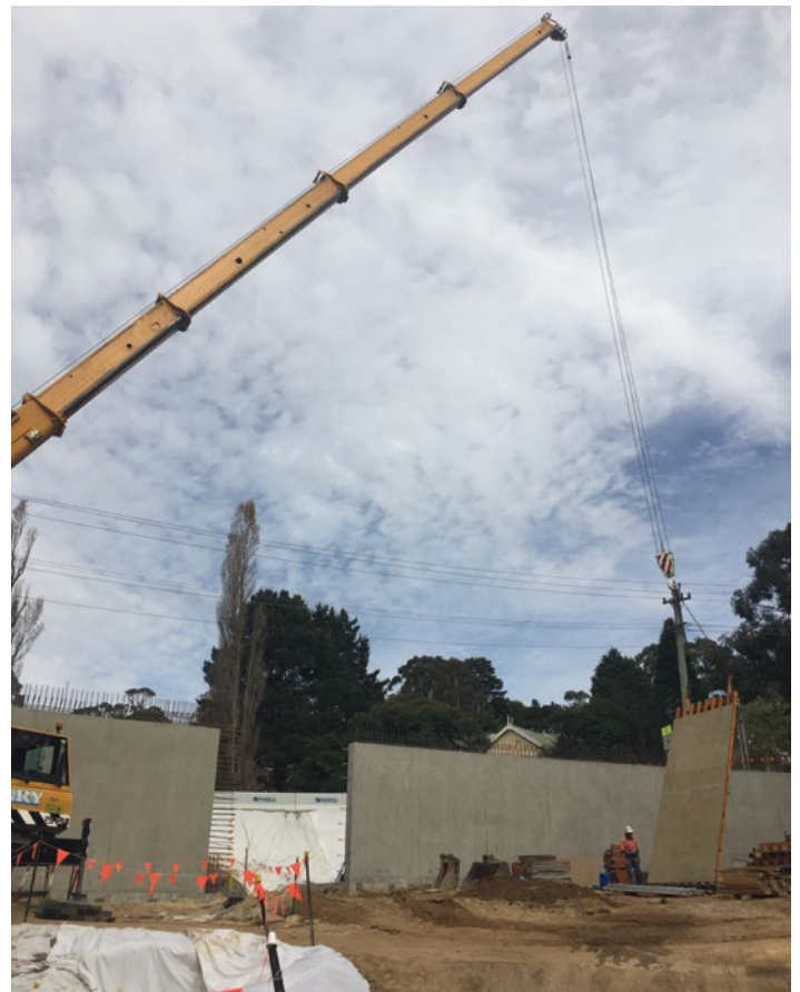
A 5.3 m retaining wall at Mount Victoria under construction.
