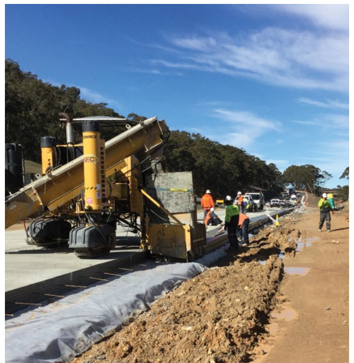
Concrete kerb pour at Forty Bends.
