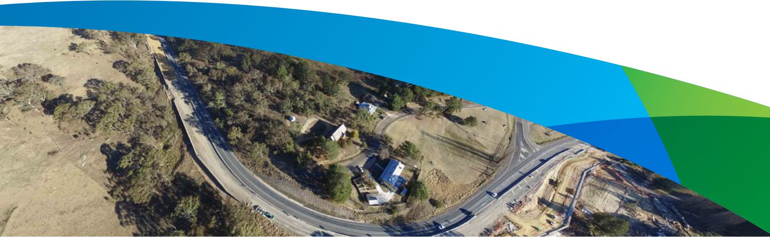
Hartley Historic Site curve, Great Western Highway. Aerial photos of Hartley Historic Site curve supplied by DIODRONE
