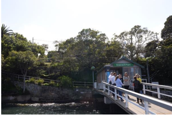
Figure 26: North-east view of the wharf at the base of the escarpment looking up towards Lower Serpentine Road
