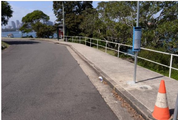
Figure 30: South-east view of Lower Serpentine Road, with no sandstone elements present
