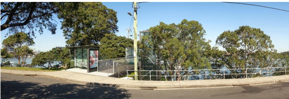
Figure 48: View of proposal looking south from Lower Serpentine Road (provided by Transport for NSW)
