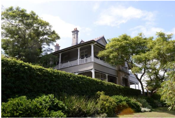
Figure 42: West view of 'Toora', House (LEP no. I110), from Lower Serpentine Road
