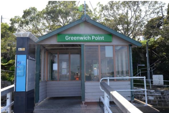
Figure 36: North-east view of the ferry shelter from the wharf ramp
