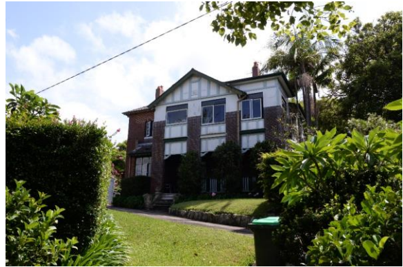
Figure 43: North-west view of 'Buena Vista', House (LEP no. I111), from Mitchell Street
