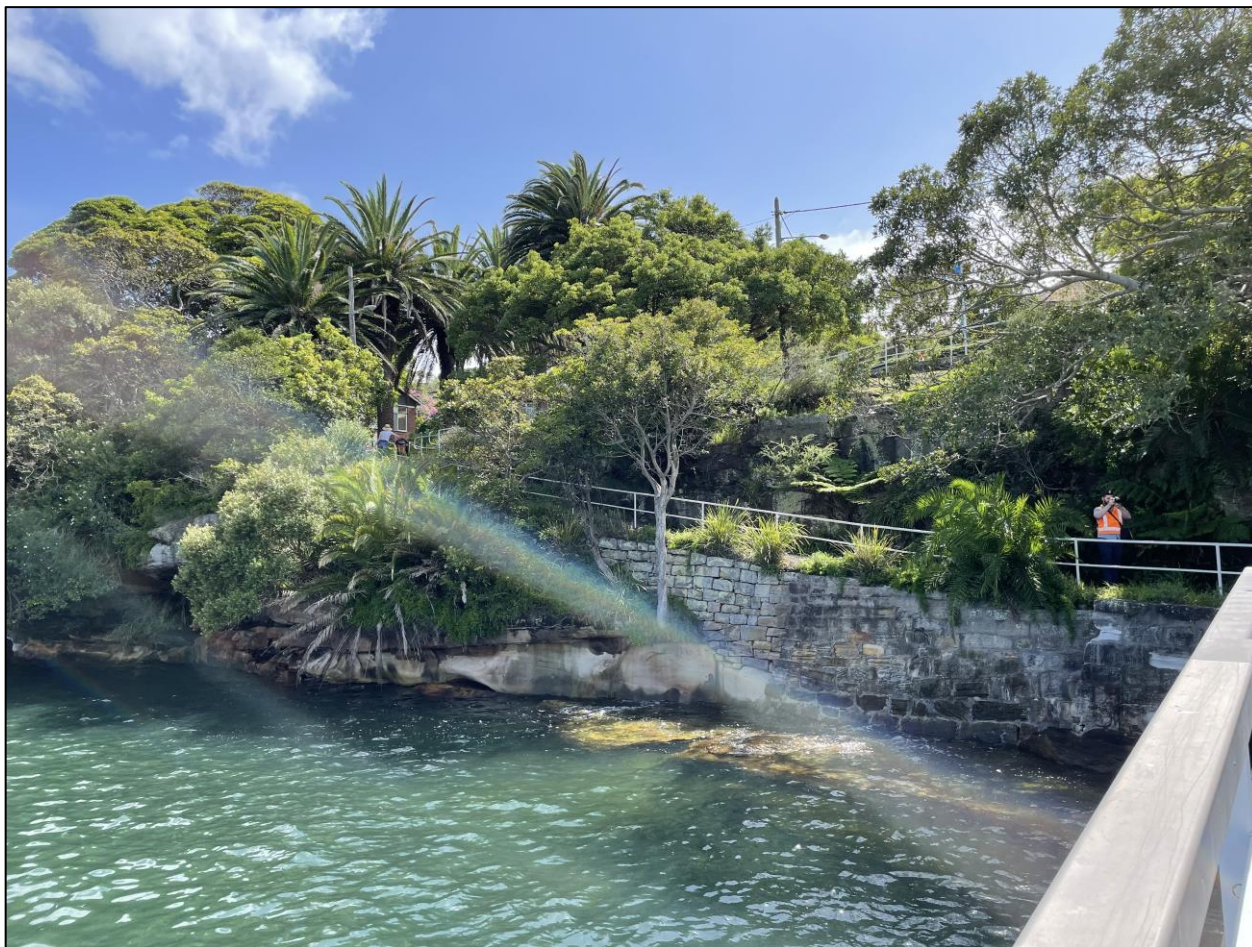
Photograph 1: Facing north-west from the wharf to the landside portion, sea wall and vegetation present.
