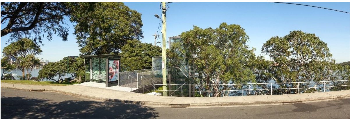
Figure 48: View of proposal looking south from Lower Serpentine Road (provided by Transport for NSW)
