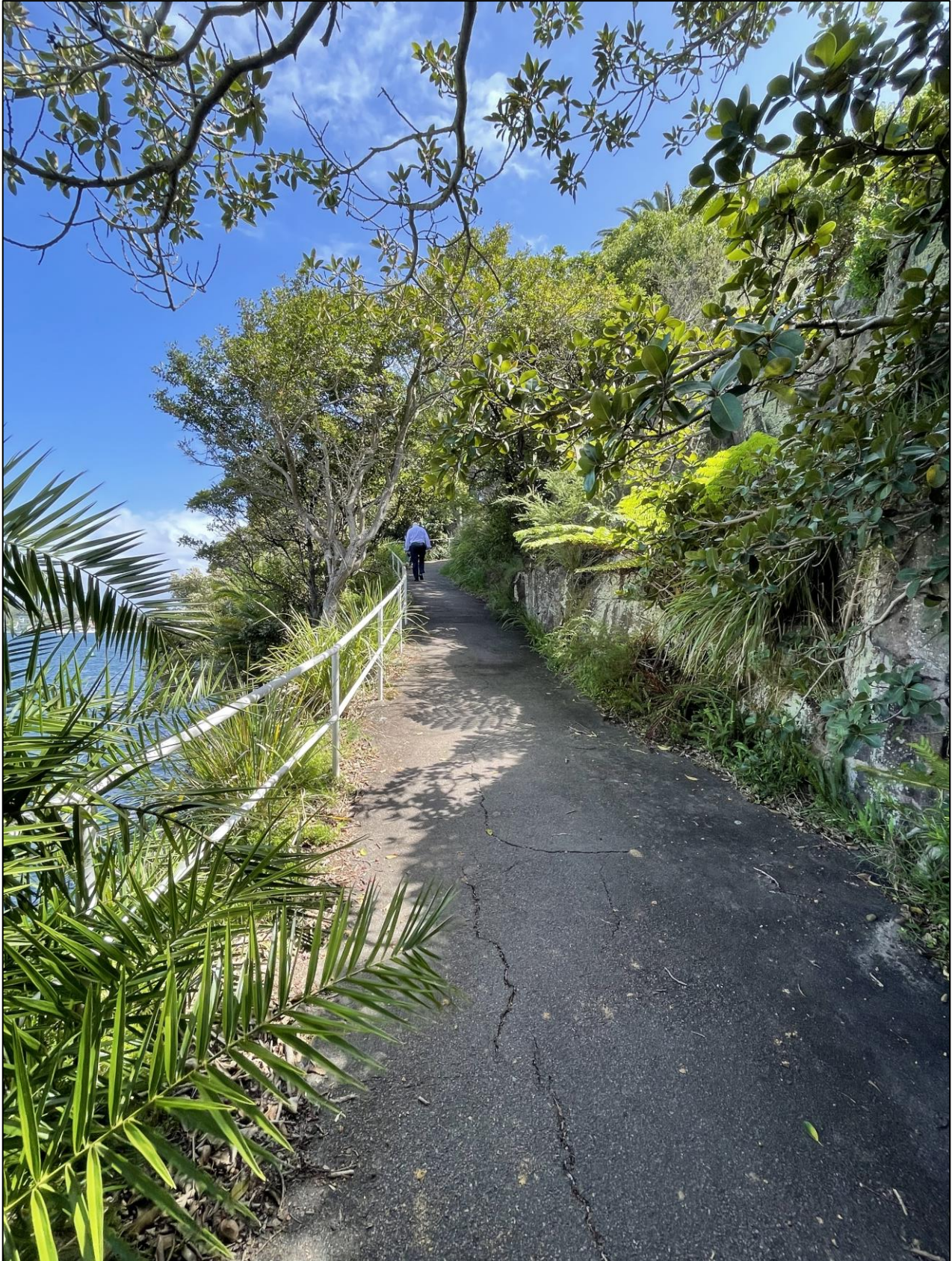
Photograph 3: Facing west, footpath and vegetation connecting Greenwich Point wharf and the footpath, some cracks evident in hardstand surface.
