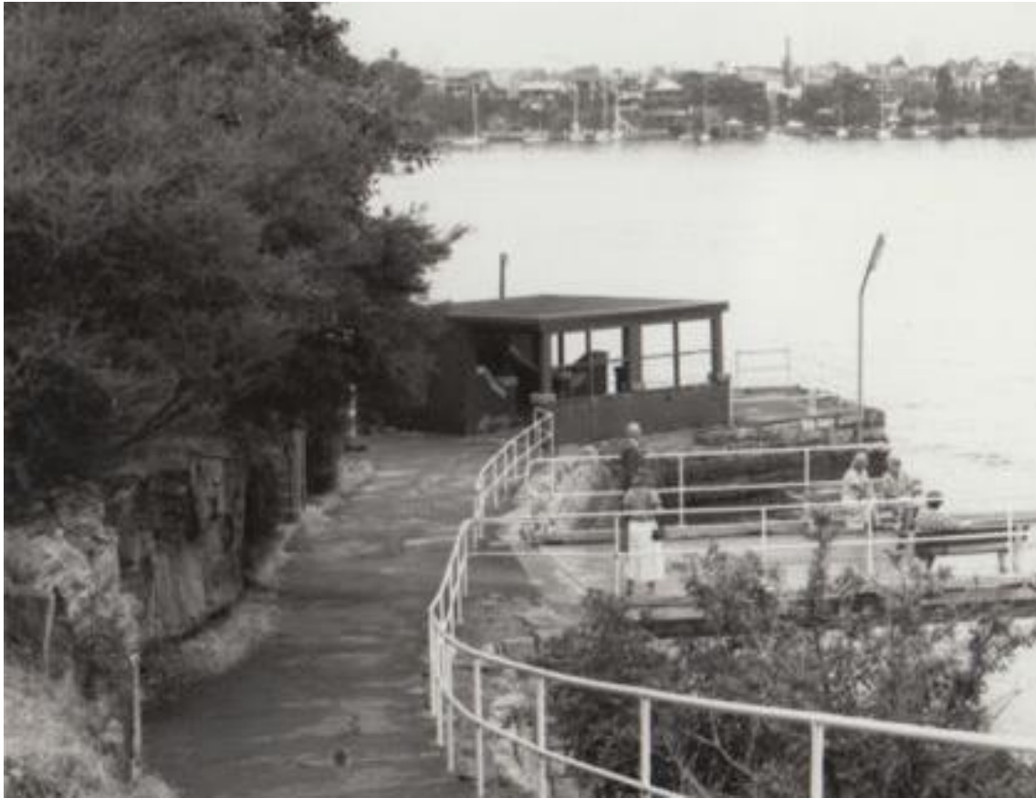
Figure 23: A 1987 view when identified for heritage listing. Source: Lane Cove Council via SHI
