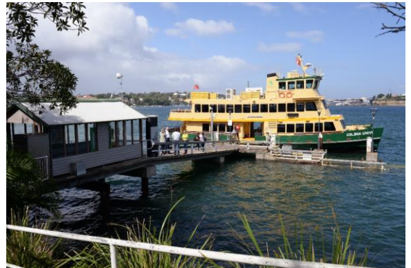
Figure 31: South view of the Greenwich Point Wharf in use
