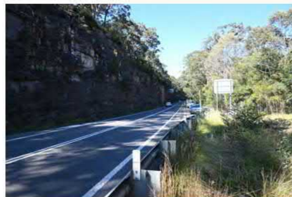
View 04 Sandstone cutting at the southern approach creates a visually dramatic setting and displays the rugged topography.
