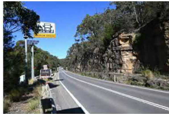
View 02 View looking south from the northern approach to the bridge. To the right side of the picture, sandstone cuttings expose the geology of the area.
