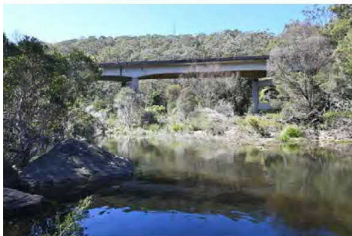
Figure 15. View of existing bridge looking east
