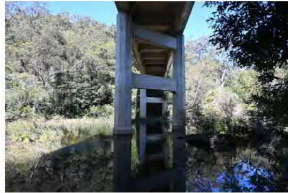
View 06 View looking north from beneath the structure.
