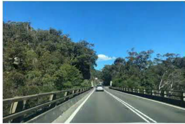
View 03 Crossing over the Woronora River with panoramic vistas of the pristine bushland.
