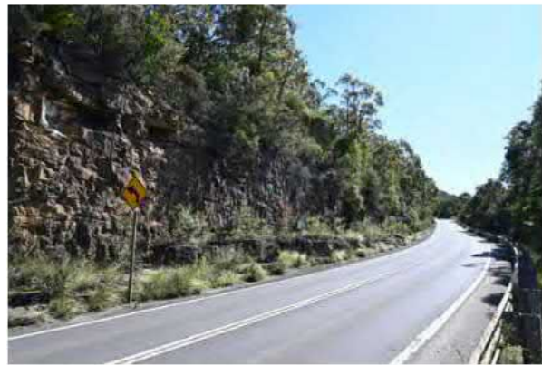
View 01 View looking north near the northern approach to the bridge.
