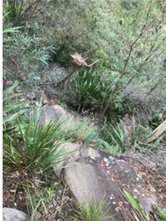
Figure 35: Sandstone chute which drains flow from outlet, provided by Fulton Hogan.
