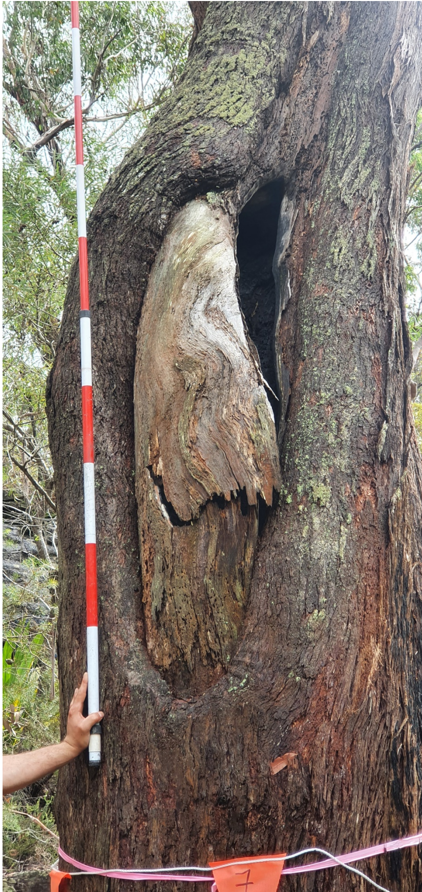
Site photo: Heathcote Road bridge, vegetation above north-west cutting
