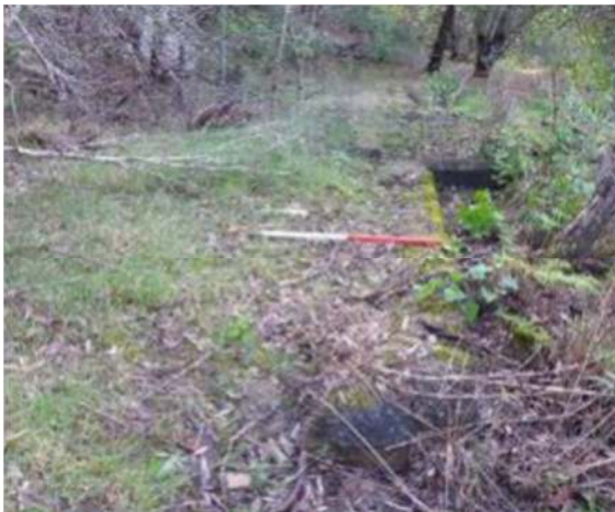
Figure 24: Concrete foundations located in the north-western portion of the study area, most likely associated with the Kolora Weir and the amenities block (Source: Biosis, 2020).
