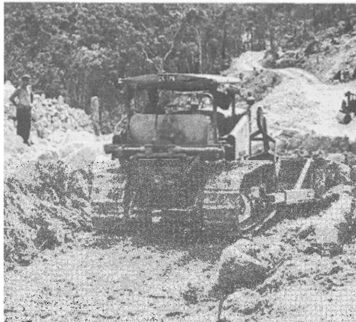
Figure 18: Construction of Heathcote Road, 1941 (Source: Department of Main Roads, NSW, 2000).
