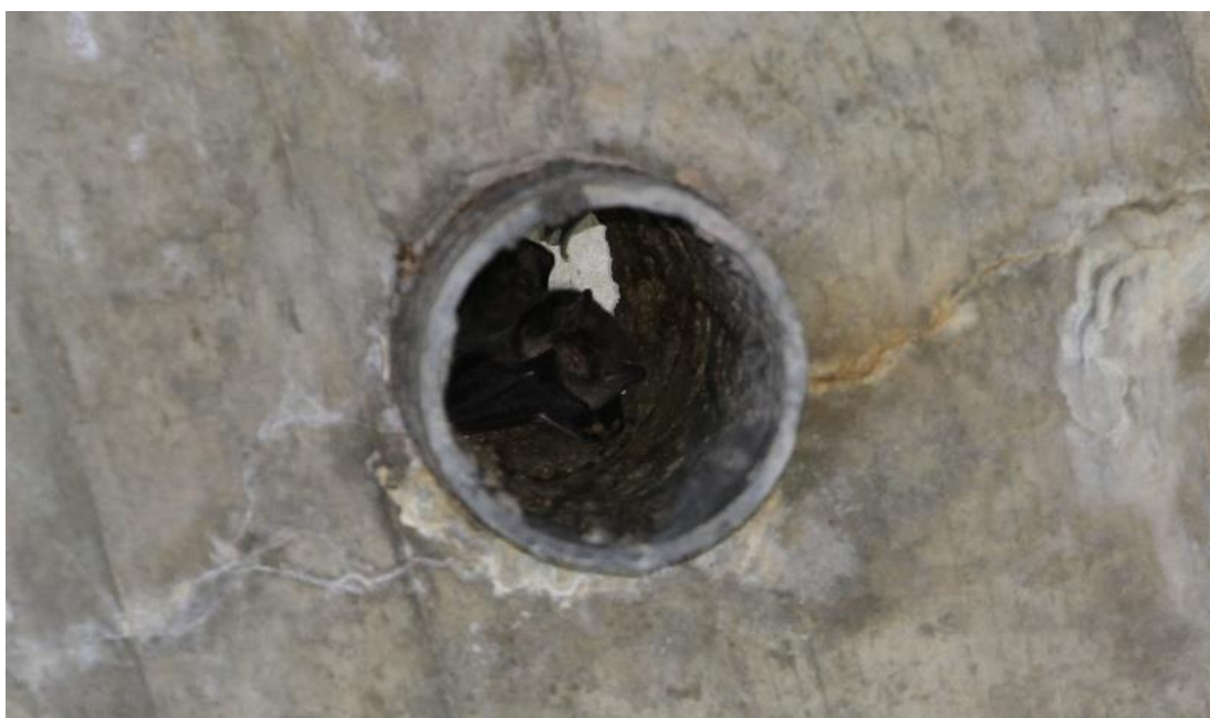
Figure 3-8 Southern Myotis in bridge scuppers (September 2020)
