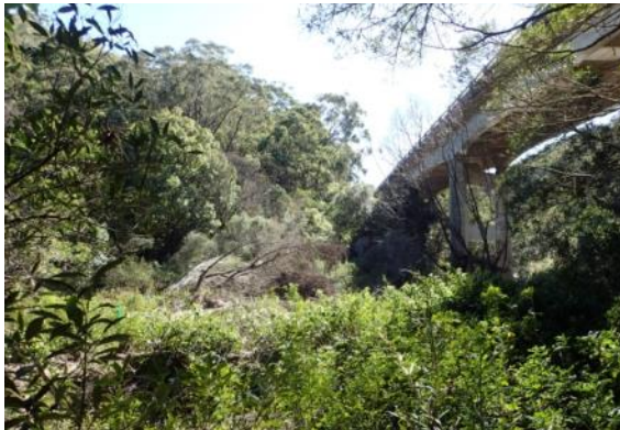
Plate 5. View to north, south of Heathcote Road Bridge over Woronora River. Note limited surface visibility due to dense vegetation and weed covered sandbars.
