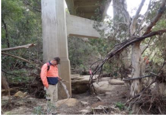
Plate 11. Photo of bridge abutment flat sandstone exposures present in riverbed.
