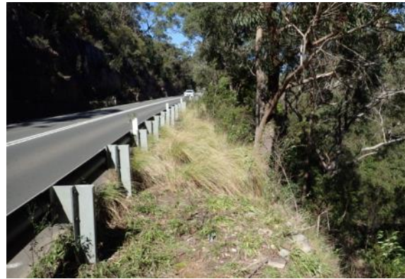
Plate 8. View south of bridge. Photo displays the top of embankment and access track. Note poor visibility and existing disturbance from previous road construction.
