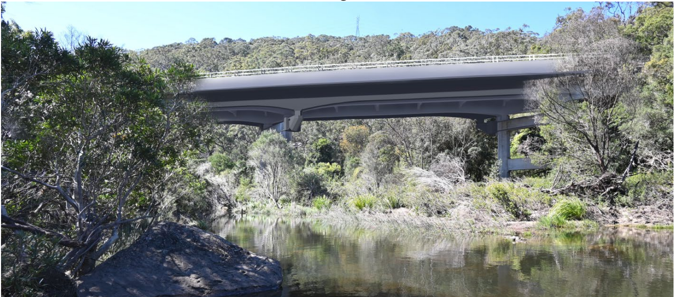
Photo 43 Photomontage of detailed concept design of Option C bridge widening (Source: TfNSW, provided 20 October 2020)
