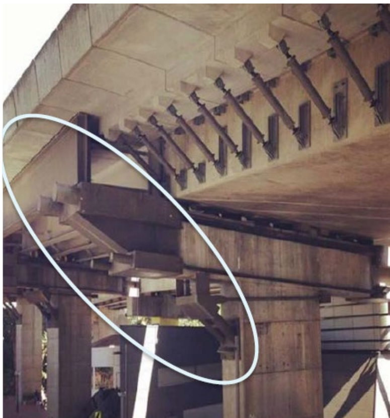
Photo 40 Example of headstock extension used for Market Street Viaduct, Darling Harbour
