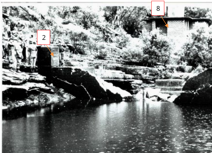
Members of the 17 th Construction squad discuss the next phase of demolition just after breaching the weir wall. Amenities block can be seen at right rear. Photo courtesy of Sutherland Library Local History section.
