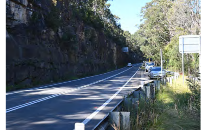
Figure 2.20 The southern approach is defined by large sandstone cuttings contributing to the scenic quality of the road.
