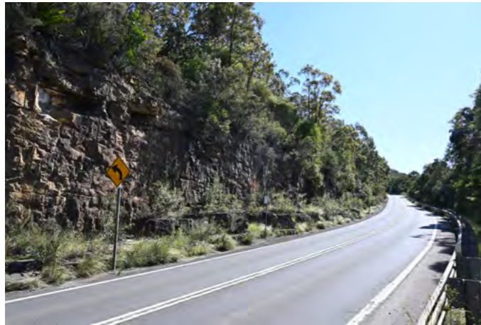
Figure 6.4 V01: View looking north near the northern approach to the bridge.
