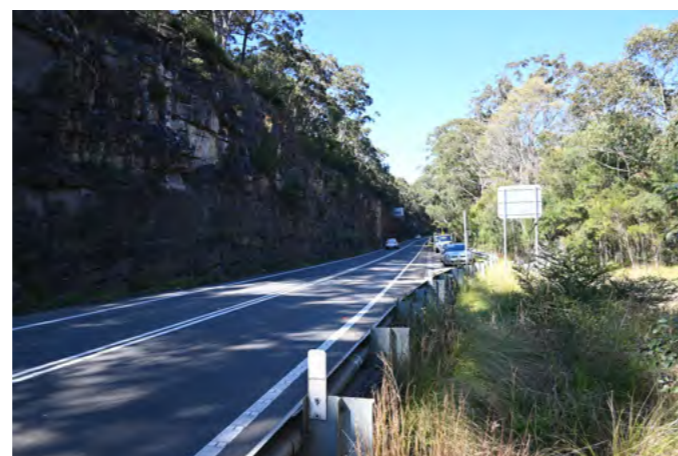
Figure 6.7 V04: Sandstone cutting at the southern approach creates a visually dramatic setting and displays the rugged topography.
