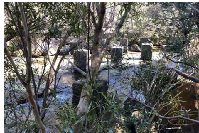
Figure 2.11 Remnants of the old piers of the original river crossing.
