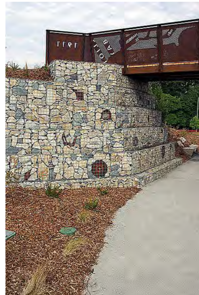
Figure 5.10 This example uses larger size rock. However, this will impact the basket's width.
