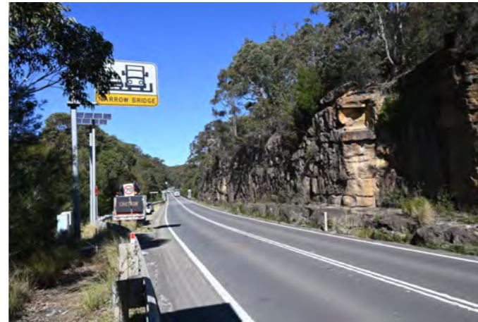
Figure 6.5 V02: View looking south from the northern approach to the bridge. To the right side of the picture, sandstone cuttings expose the geology of the area.
