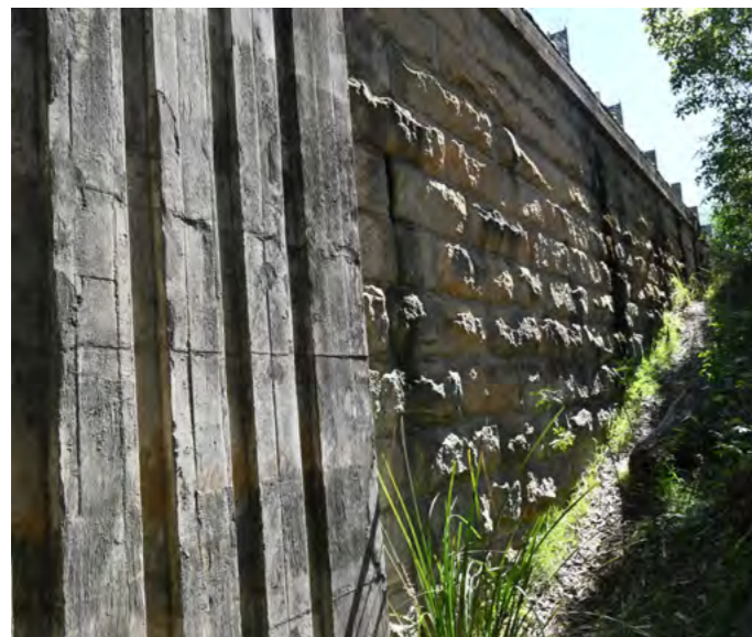
Figure 5.8 Existing abutment return wall showing the sandstone cladding.
