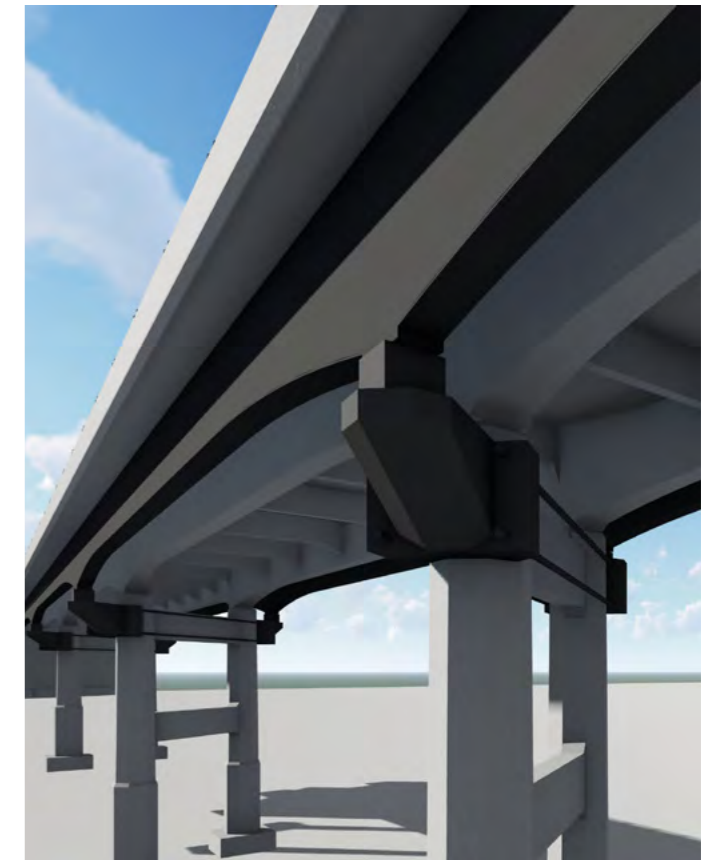
Figure 5.5 Indicative 3D study of the girder, illustrating the haunched form language at the pier.
