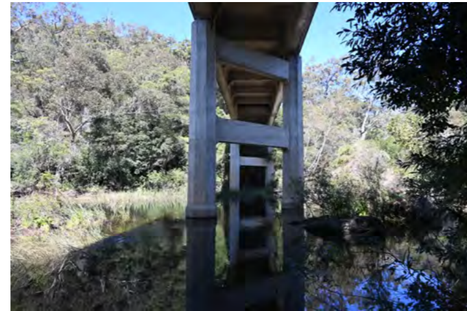
Figure 6.9 View looking north from beneath the structure.
