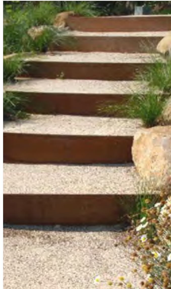
Figure 5.15 Example of a stair using weathered steel risers and stabilised gravel treads.
