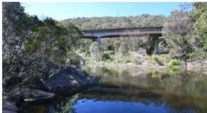
Figure 5.21 View of the existing bridge looking east.
