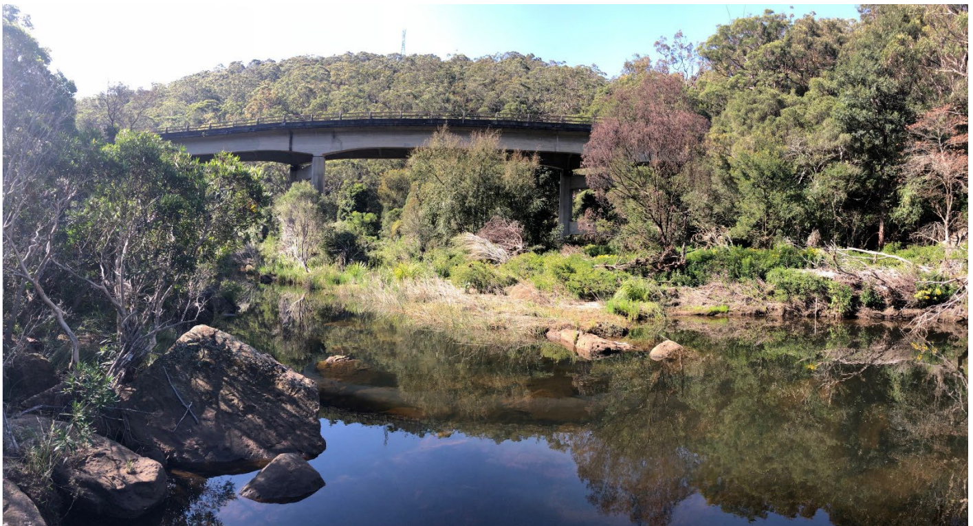
Existing Heathcote Road Bridge
