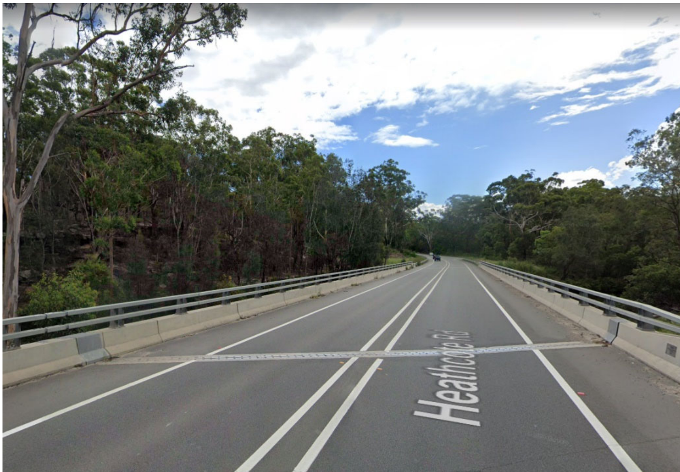
Figure 3-2 Example of a similar bridge structure at Deadmans Creek bridge
