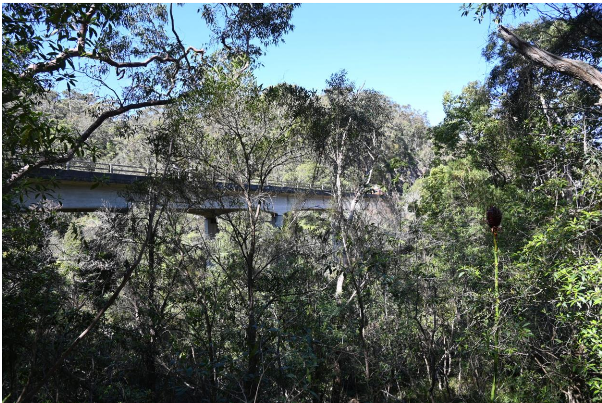
Figure 6-30 View looking towards the existing bridge showing screening effect of bushland
