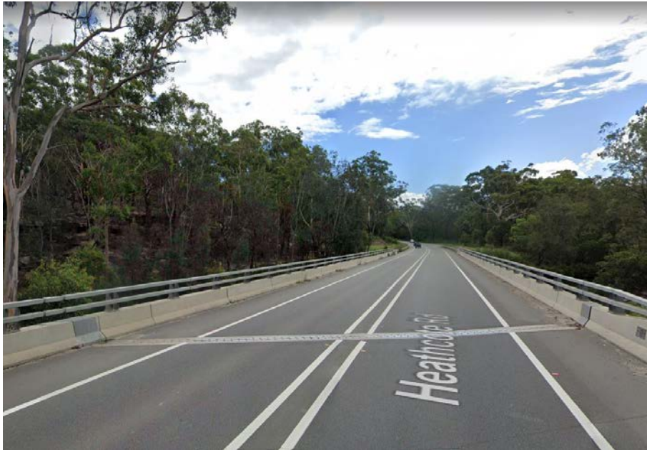
Figure 2-7 Example of a similar bridge structure at Deadmans Creek bridge
