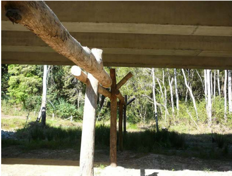
Figure 2-11 Example of fauna furniture installed under a bridge to facilitate the movement of koalas (Roads and Maritime, 2019)
