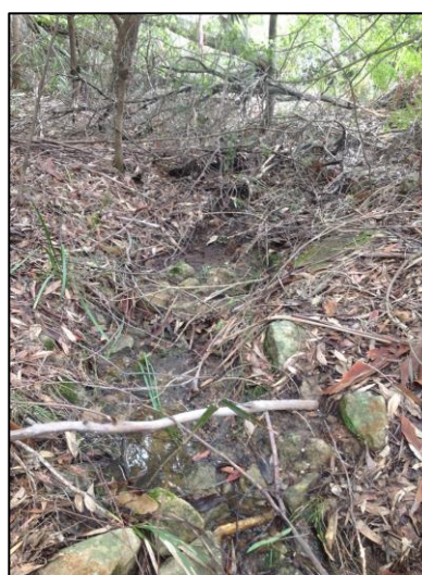
Access track, upstream on northside gully erosion and drainage (facing north)
