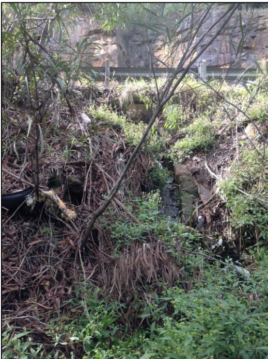
Figure 6-16 Site photo of cross drain at southern approach
