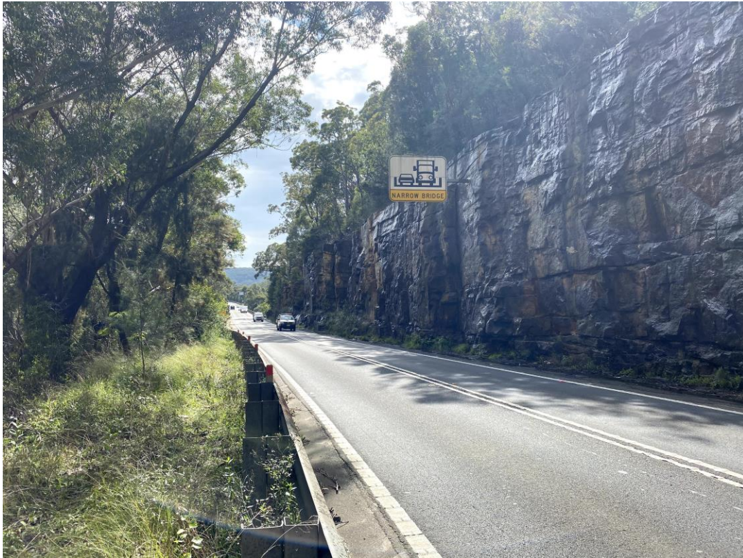
Figure 3-5 Photo showing high rock cutting and narrow lanes and shoulders on approach to the bridge
