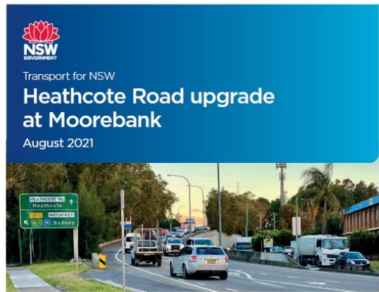
Heathcote Road at Moorebank looking south towards the M5 Motorway
