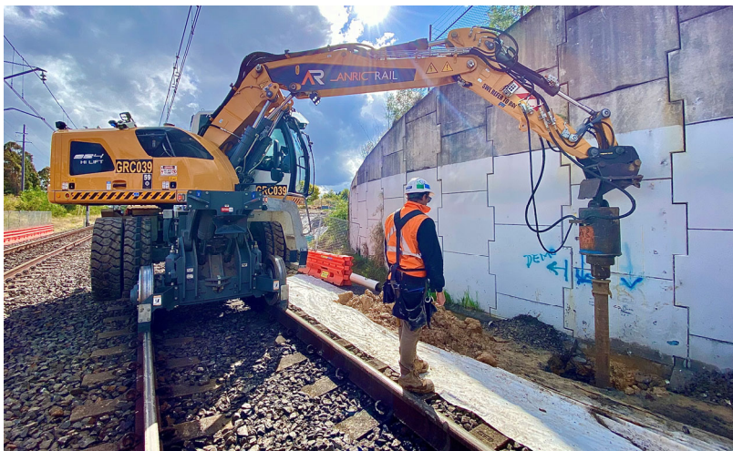
Piling works during Sydney Trains trackwork – August 2022
