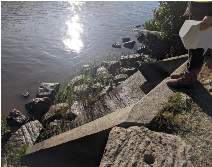
Figure 3.6 - Existing headwall and scour protection
