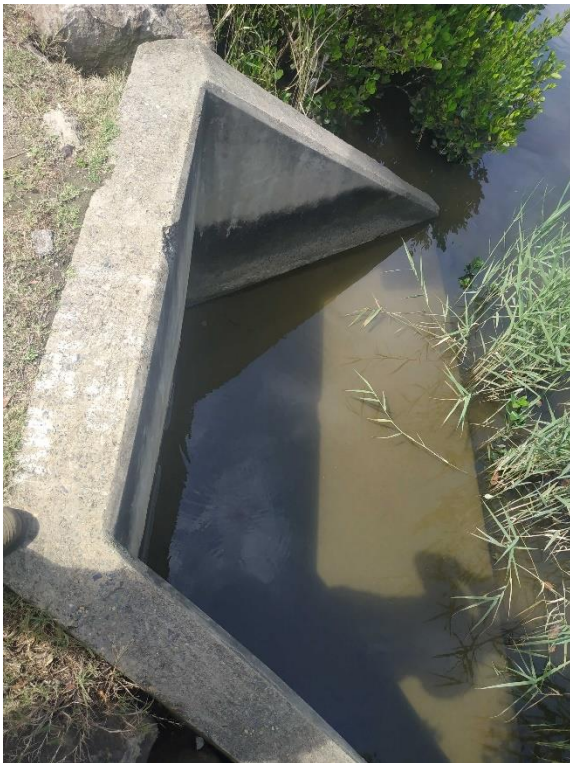
Figure 7 Headwall proposed to be replaced
