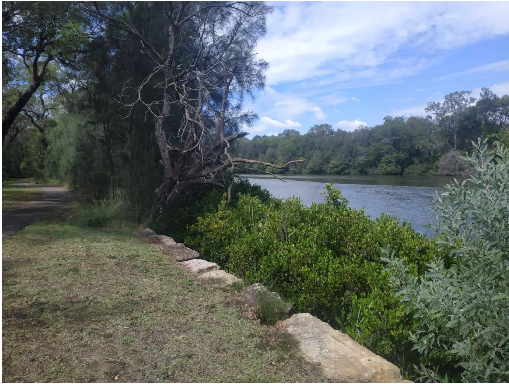
Figure 8 Riverbank in vicinity of headwall
