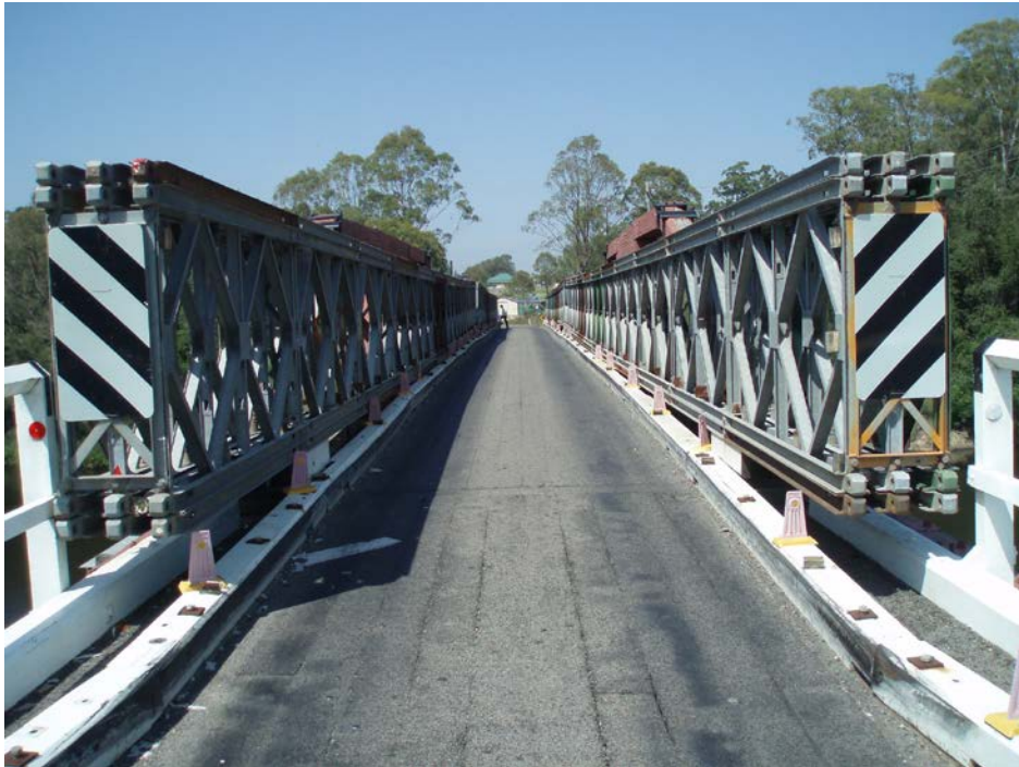
View of the bridge deck and bailey bridge structure
