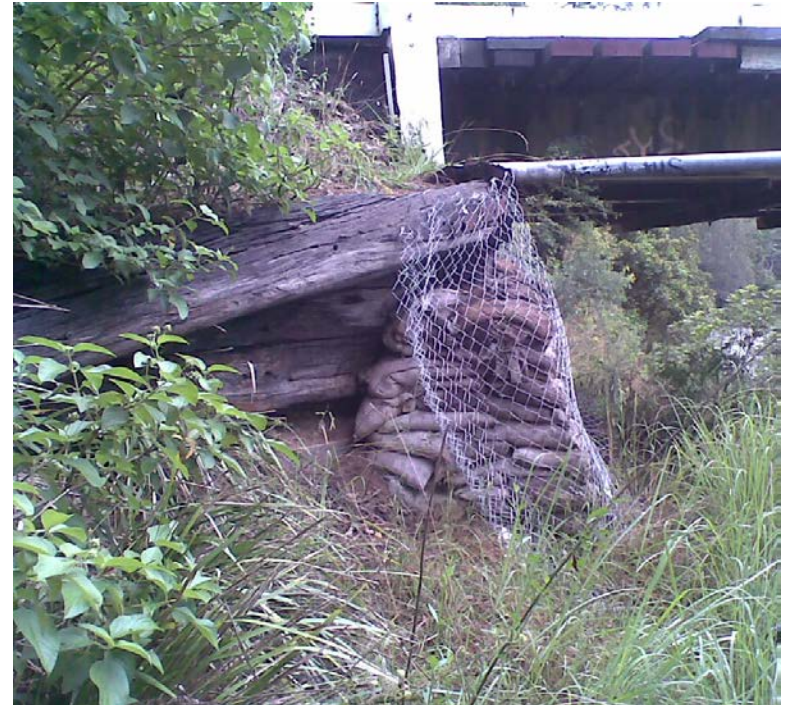
View of the current abutment
