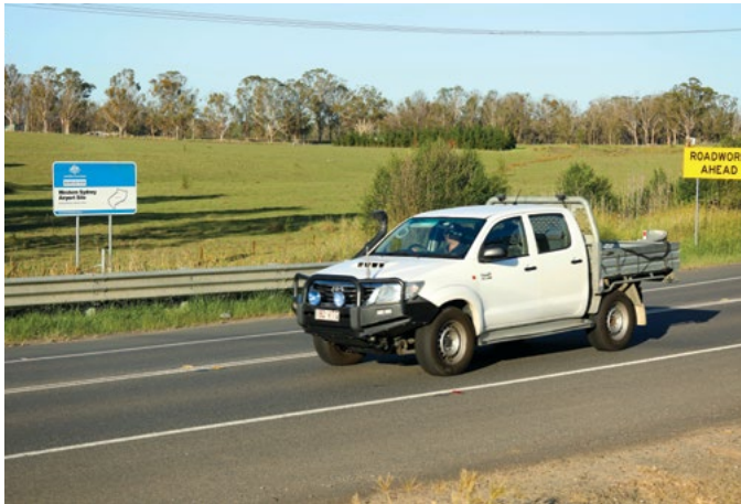
The Northern Road next to the Western Sydney Airport site
