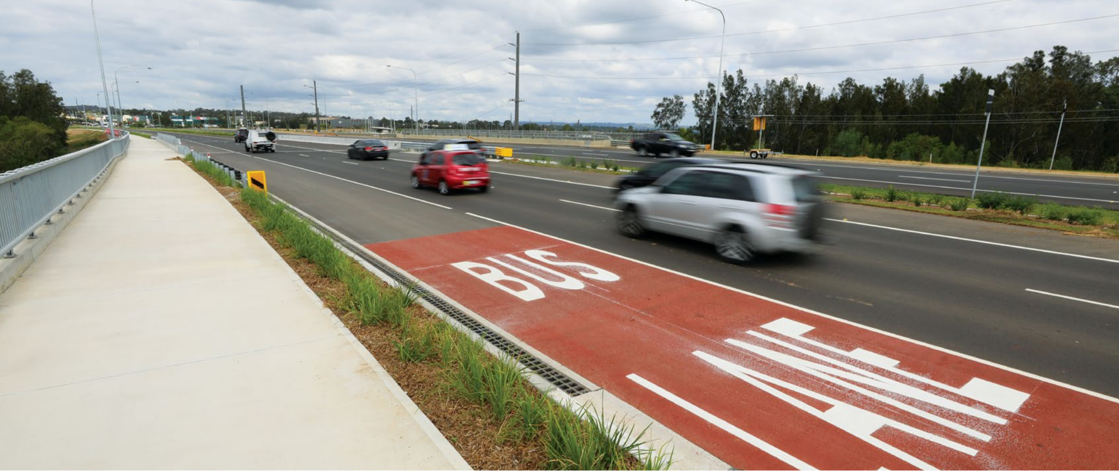
The Northern Road southbound, south of Hillside Drive
