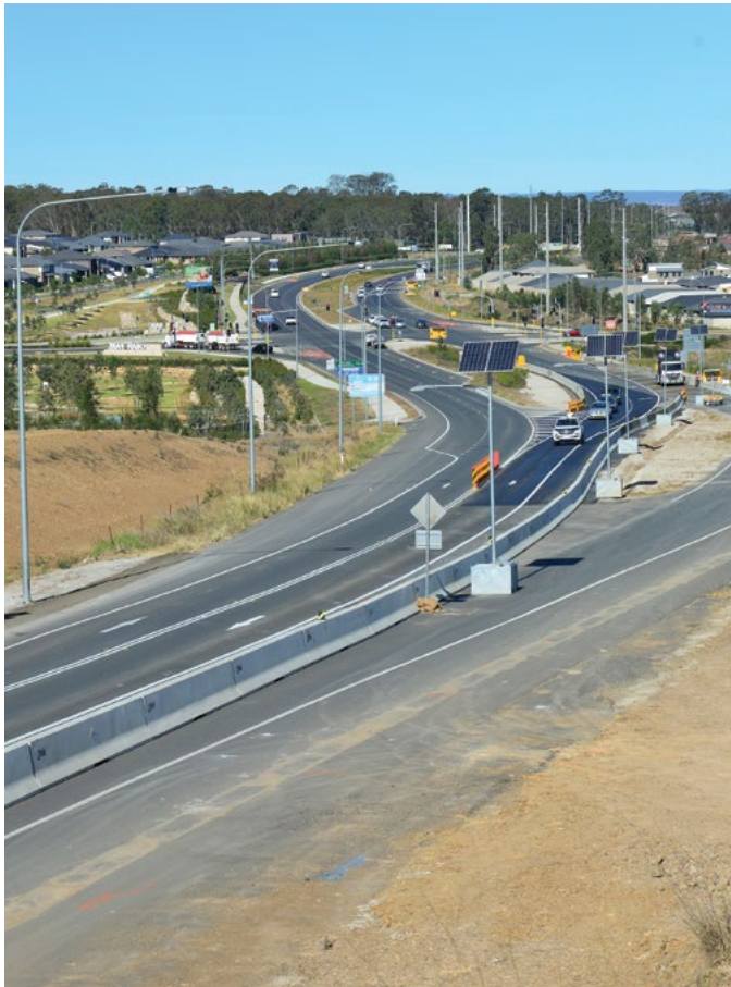
Recently completed traffic switch to facilitate the Stage 1 construction of the southern end of The Northern Road, Oran Park
