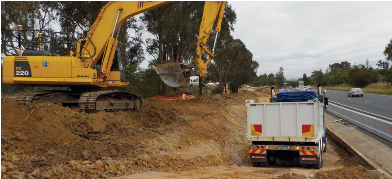
Earthwork next to the M4 Motorway, Claremont Meadows
