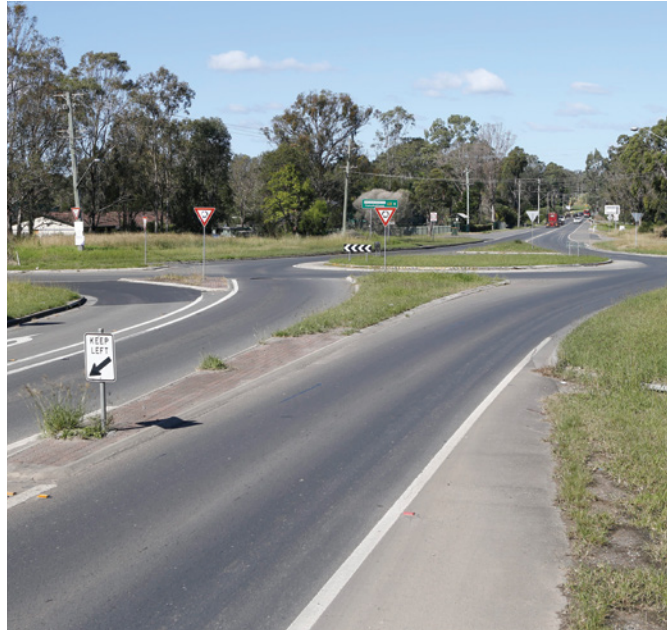
The Northern Road and Badgerys Creek intersection looking south
