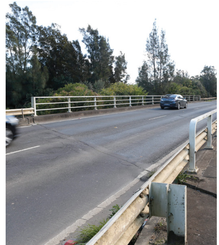
The Northern Road at the Narellan Creek Bridge looking north
