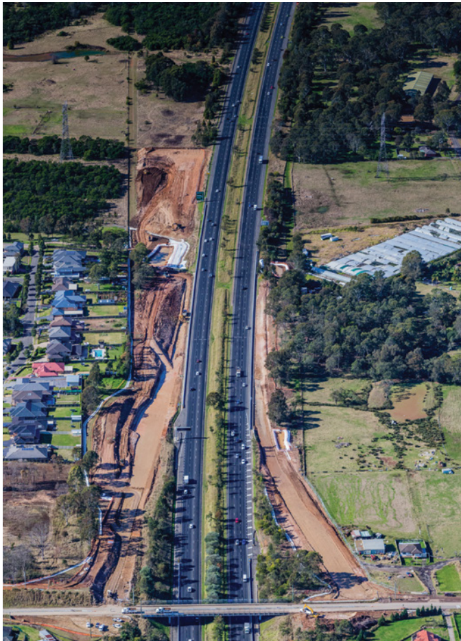
The Kent Road bridge over the M4 Motorway, Claremont Meadows
