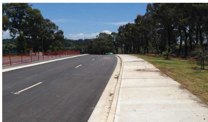
New pavement and shared path at Eagle Vale Drive
