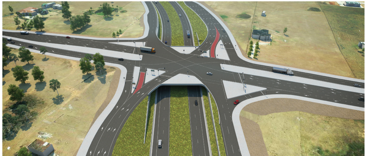
Artist impression of the proposed grade separated interchange (underpass) at The Northern Road and Bringelly Road
