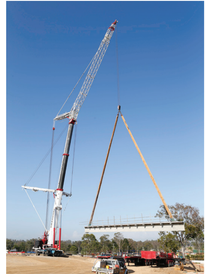
Installing a new bridge girder over canal, Bringelly Road
