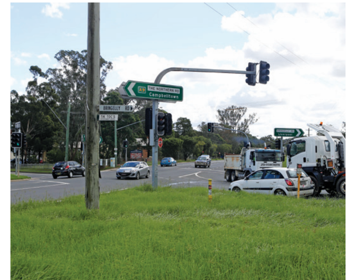
The Northern Road, Bringelly Road and Greendale Road intersection
