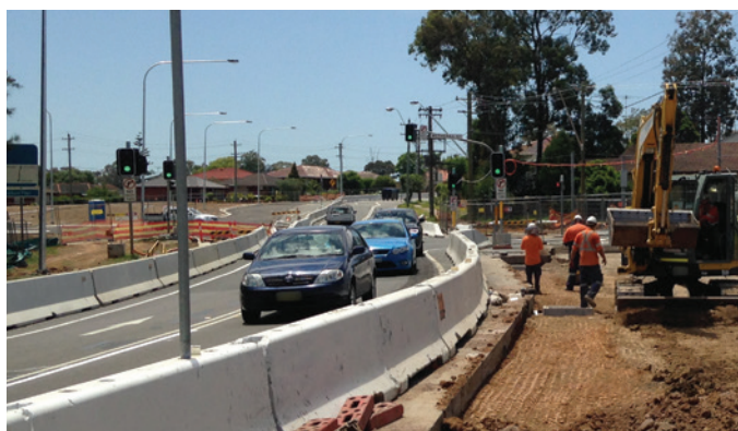
Installing drainage along The Horsley Drive, Wetherill Park
