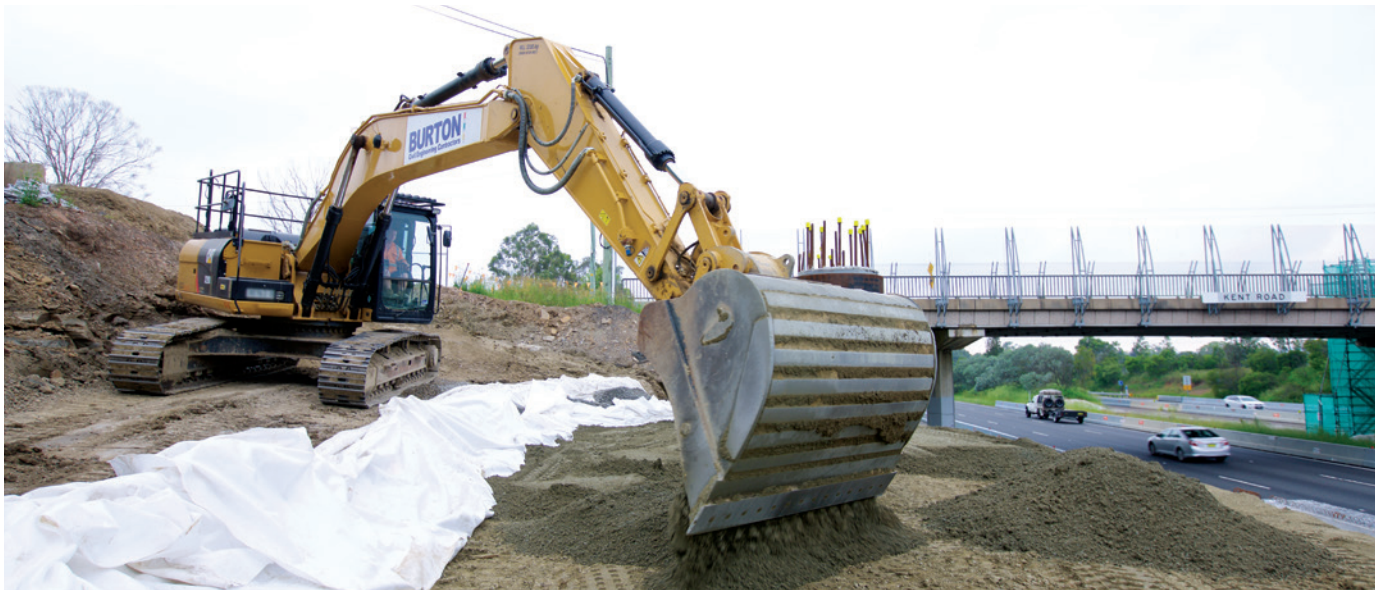
Earthwork next to the M4 Motorway, Claremont Meadows
