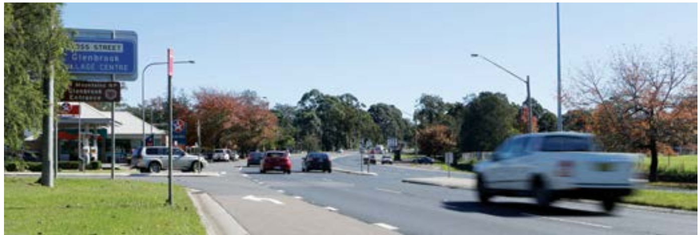
Great Western Highway and Ross Street intersection
