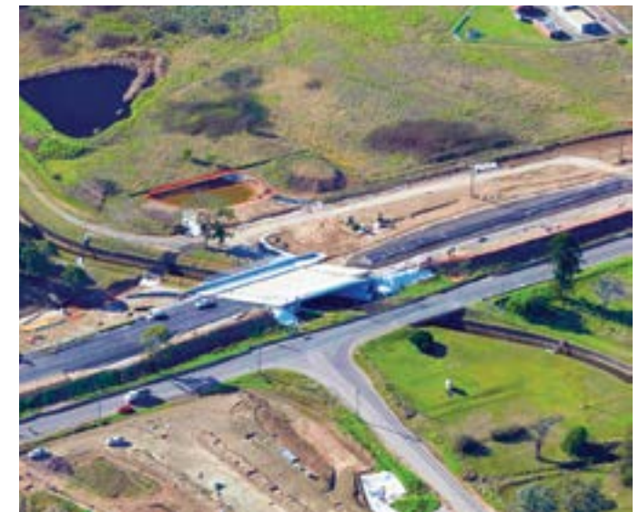
Bringelly Road, the new eastbound bridge over the WaterNSW Upper Canal
