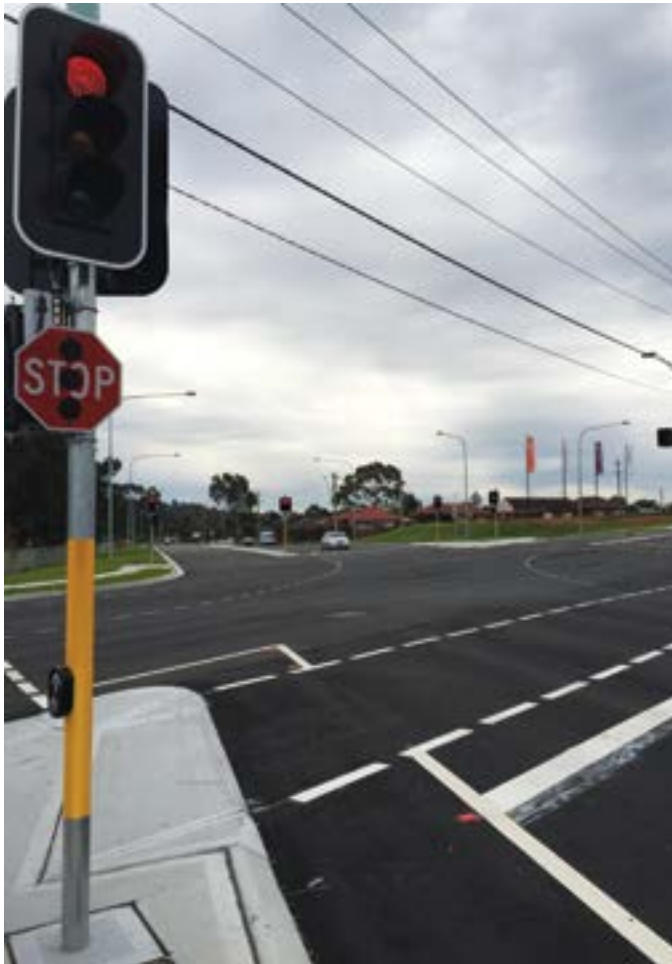
Wetherill Street Upgrade, Smithfield
