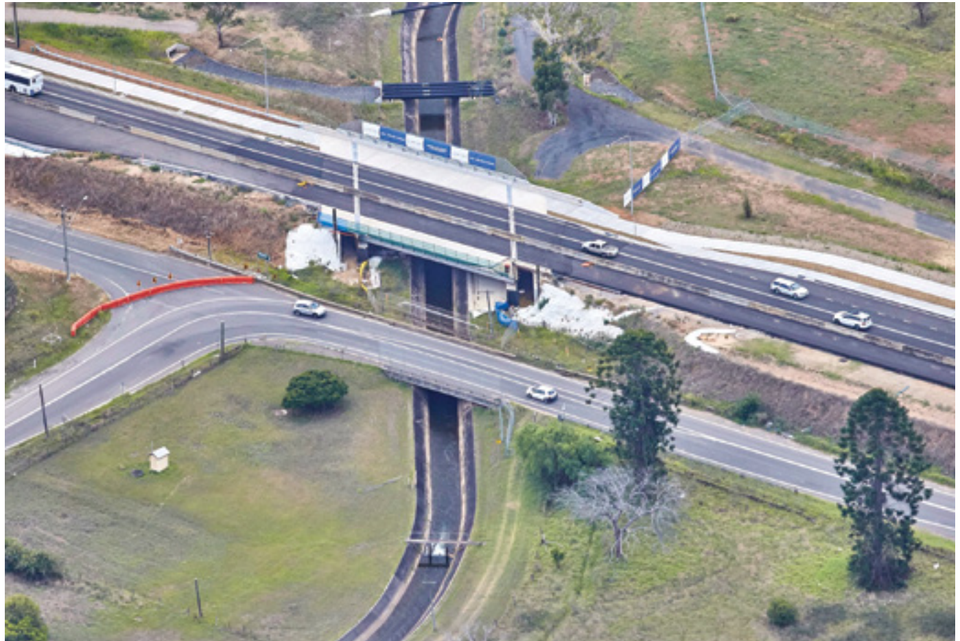
New bridge over Upper Canal on Bringelly Road Stage 1, February 2017
