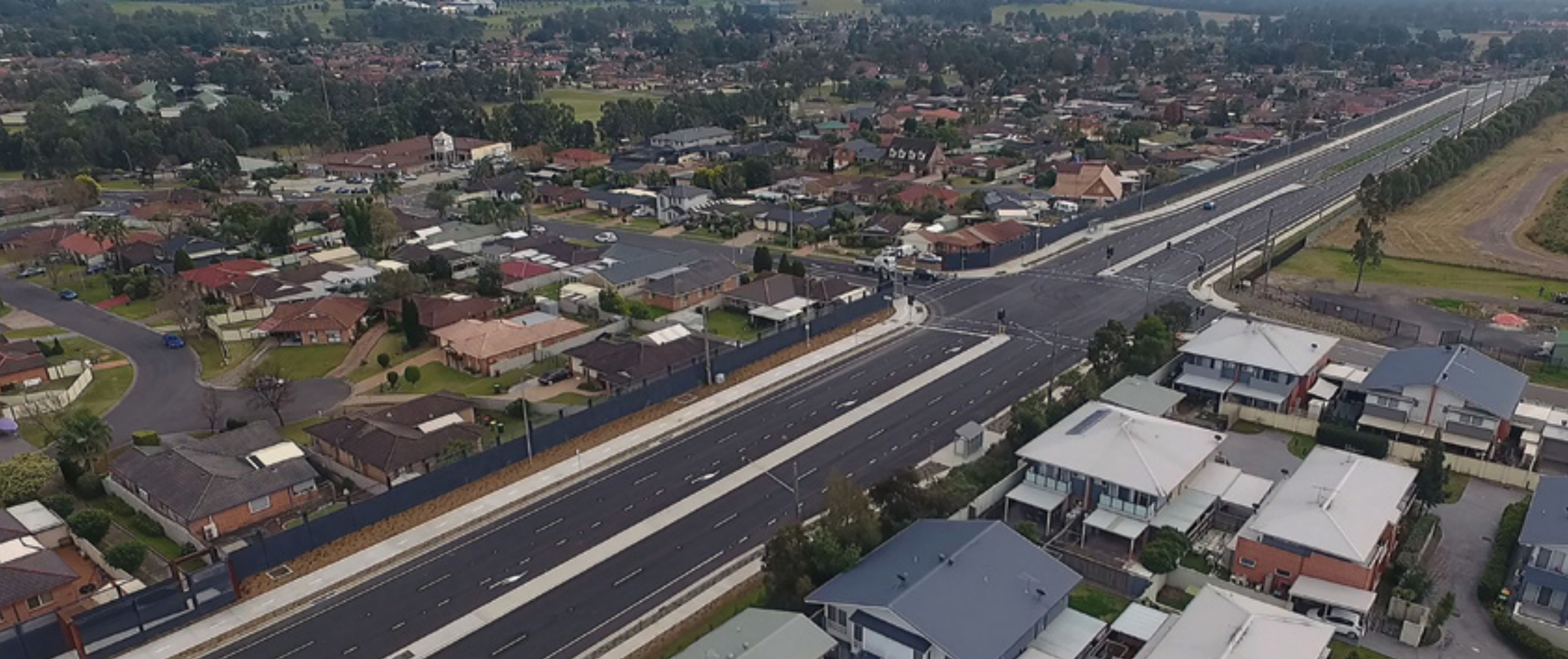
Newly built Werrington Arterial Road
