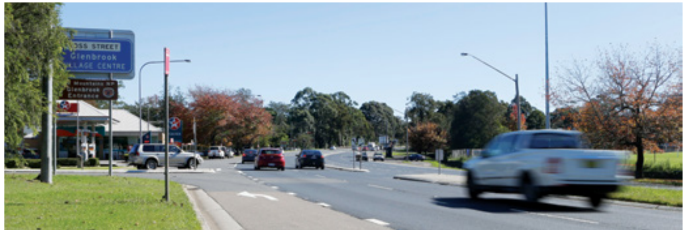
Great Western Highway and Ross Street intersection
