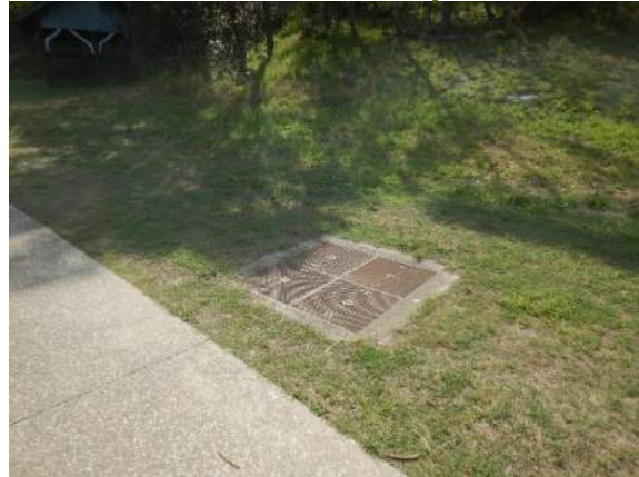
Figure 5.41: View northeast of utility vault
