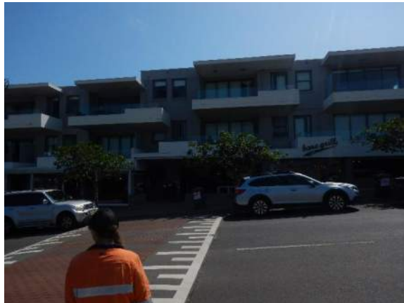
Figure 5.15: View north of buildings located in the northern portion of survey unit 3
