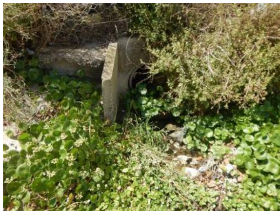
Figure 5.13: View south of drainage established within survey unit 2, below the plateau
