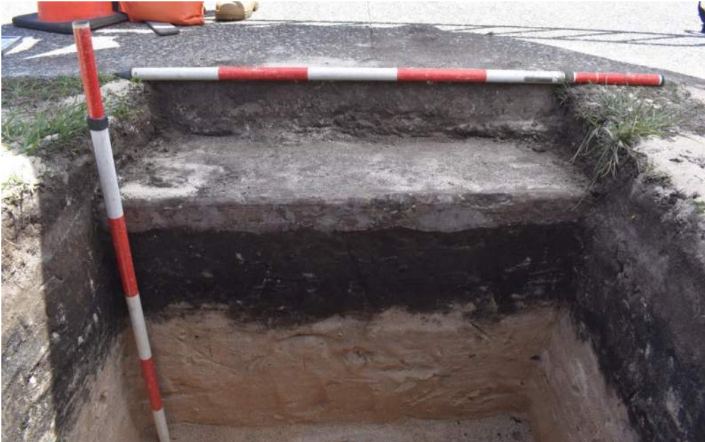
Figure 45: Profile view of the concrete slab in KU-TP22 where the concrete did not cover the entire test pit and therefore excavations were able to continue beside it
