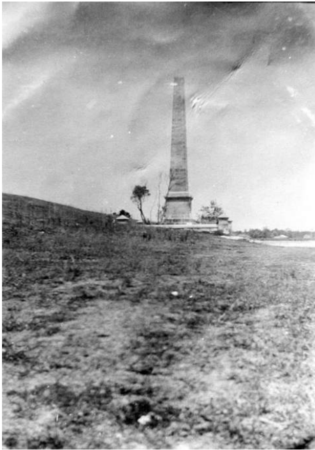
Figure 11: Photo of Cook's monument, taken around 1912. View west. Grass covered ground surface, small vegetation around Cook's monument, sandstone outcropping at front of Cook's monument
