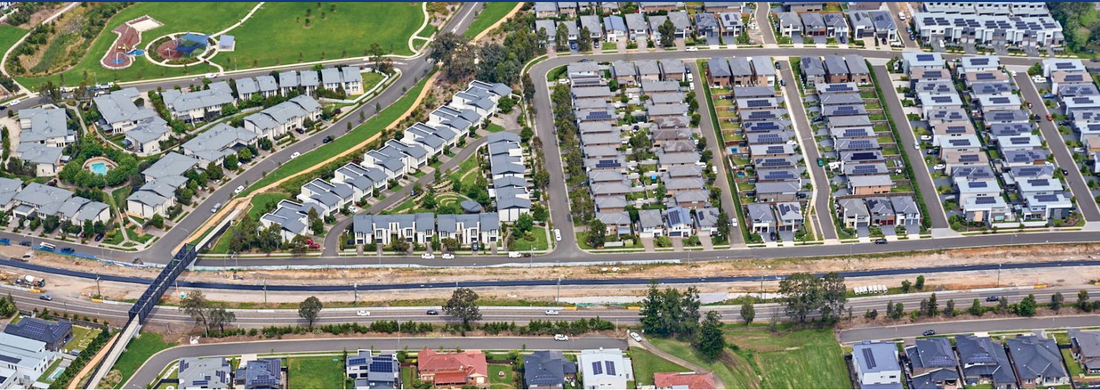
Stage 1 construction next to Rutherford Avenue – lean-mix concrete paving with asphalt curing
