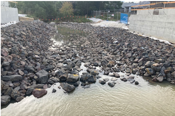
Before, without low-flow channel (facing North)
