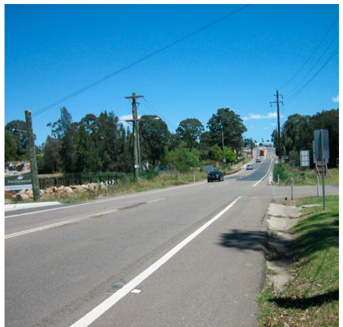
Memorial Avenue near Arnold Avenue west.
