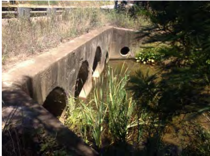
Figure 2.4 Existing culverts at Strangers Creek
