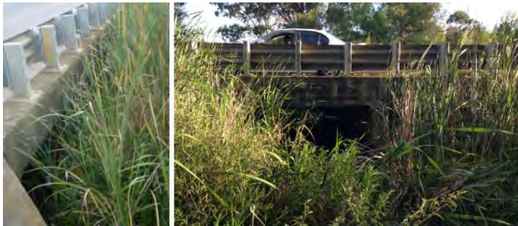
Figure 2.3 Existing culverts at Elizabeth Macarthur Creek
