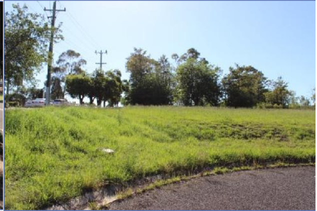
Figure 10: View east of cut, road and service infrastructure.
