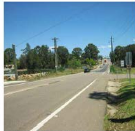
Memorial Avenue near Arnold Avenue west.
