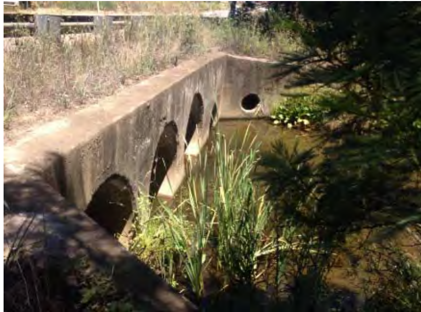
Figure 2.4 Existing culverts at Strangers Creek
