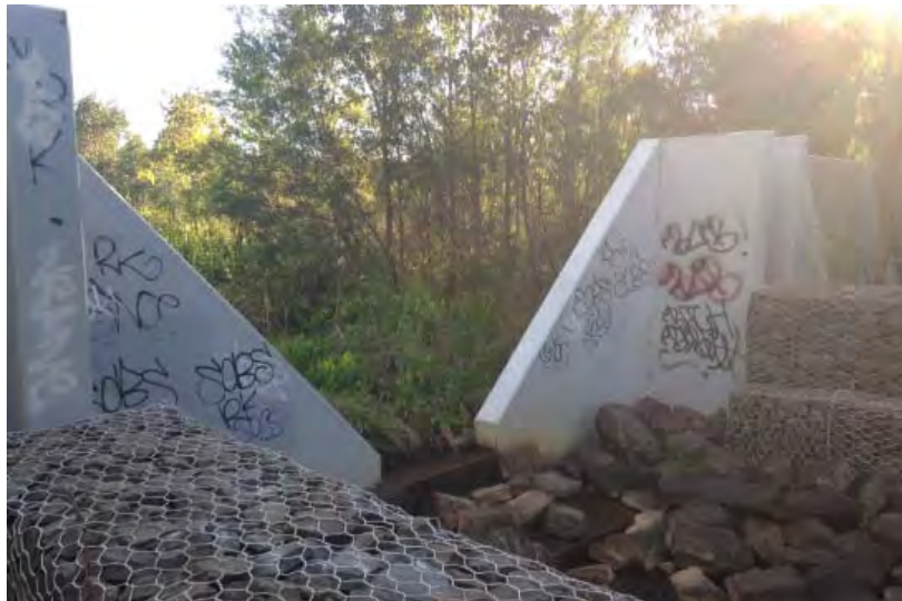
Figure 2.6 The v-notch weir structure basin outlet at Strangers Creek
