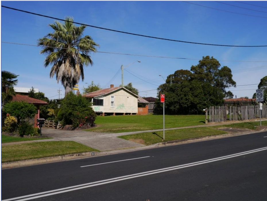
Figure 24: View south of the heritage listed property from President Avenue. Artefact Heritage 2014.
