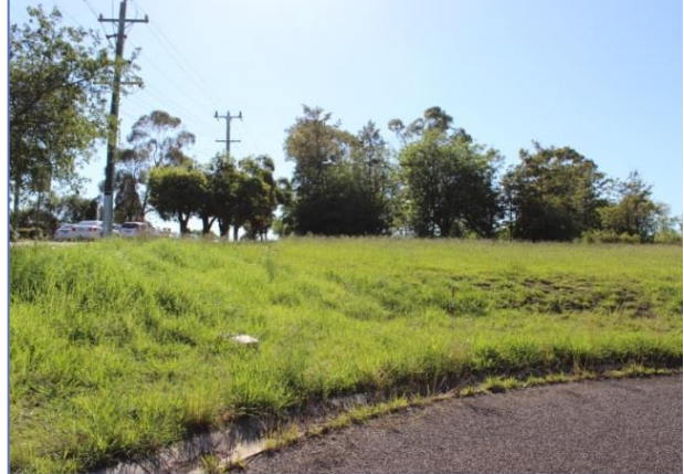
Figure 10: View east of cut, road and service infrastructure.
