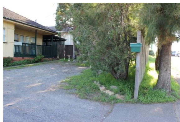
Figure 8: View east showing typical house frontage.
