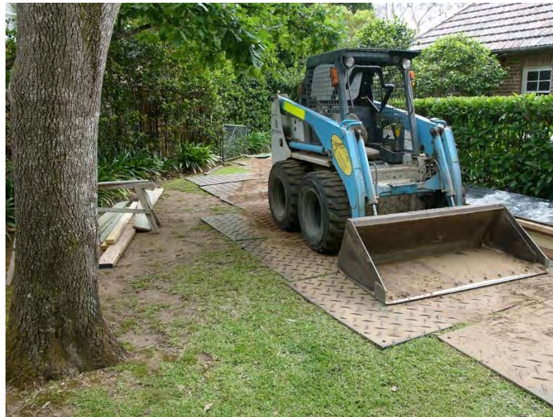
Figure 4 – Showing typical detail for truck mats.
