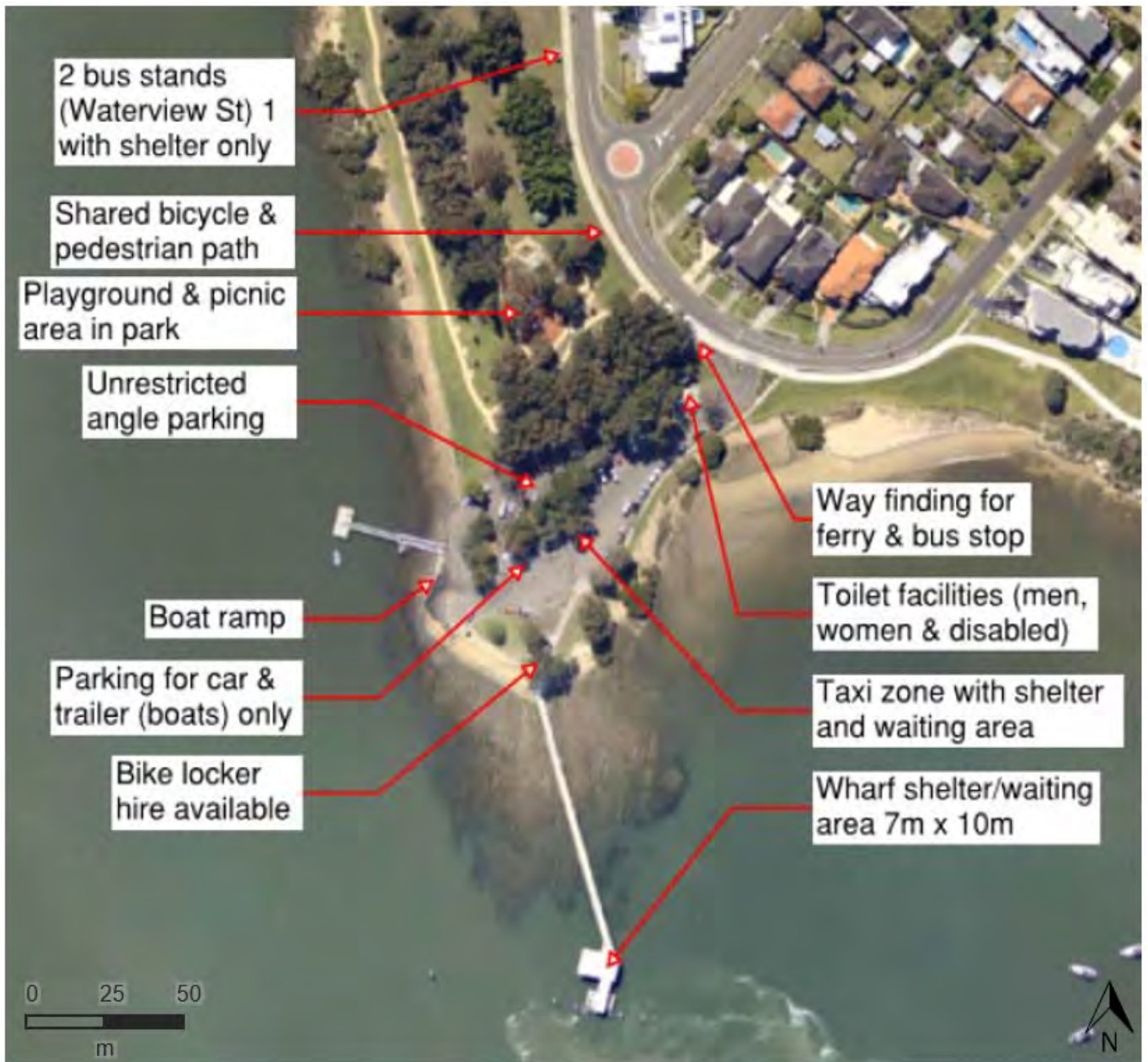
Figure 1-2 Local setting and existing infrastructure at Kissing Point Wharf
