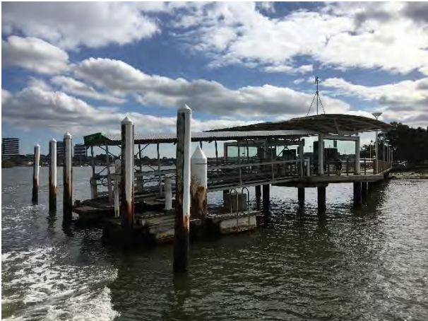
Wharf to be replaced
