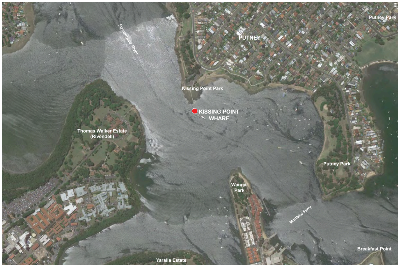
Figure 3. Existing foreshore with proposed wharf entry location (image courtesy of Google Maps)
