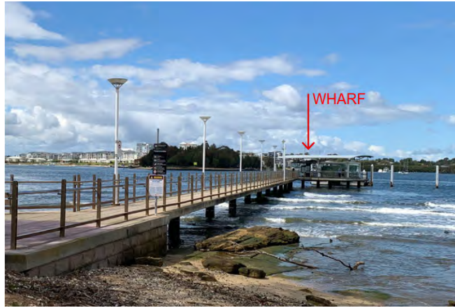
Figure 6-25 Kissing Point Wharf
