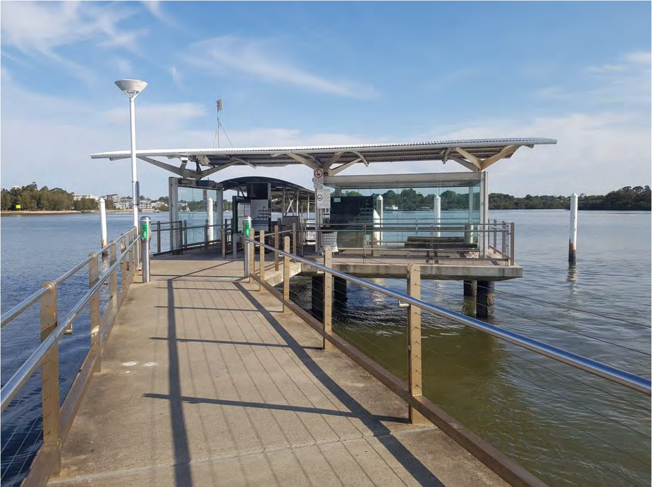
Figure 27: At the end of the jetty is a rectangular, steel-framed waiting-shelter pavilion supported on concrete piles with a shallow curved corrugated metal roof
