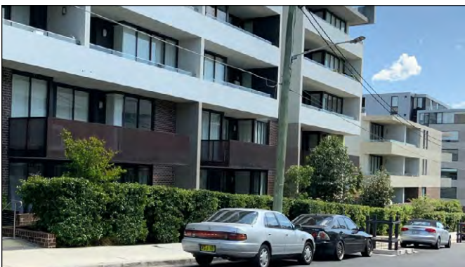
Figure 27. Character of redevelopment on Mortlake Peninsula
