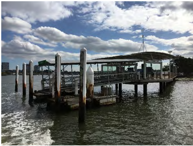
Figure 6-5 Wharf to be replaced
