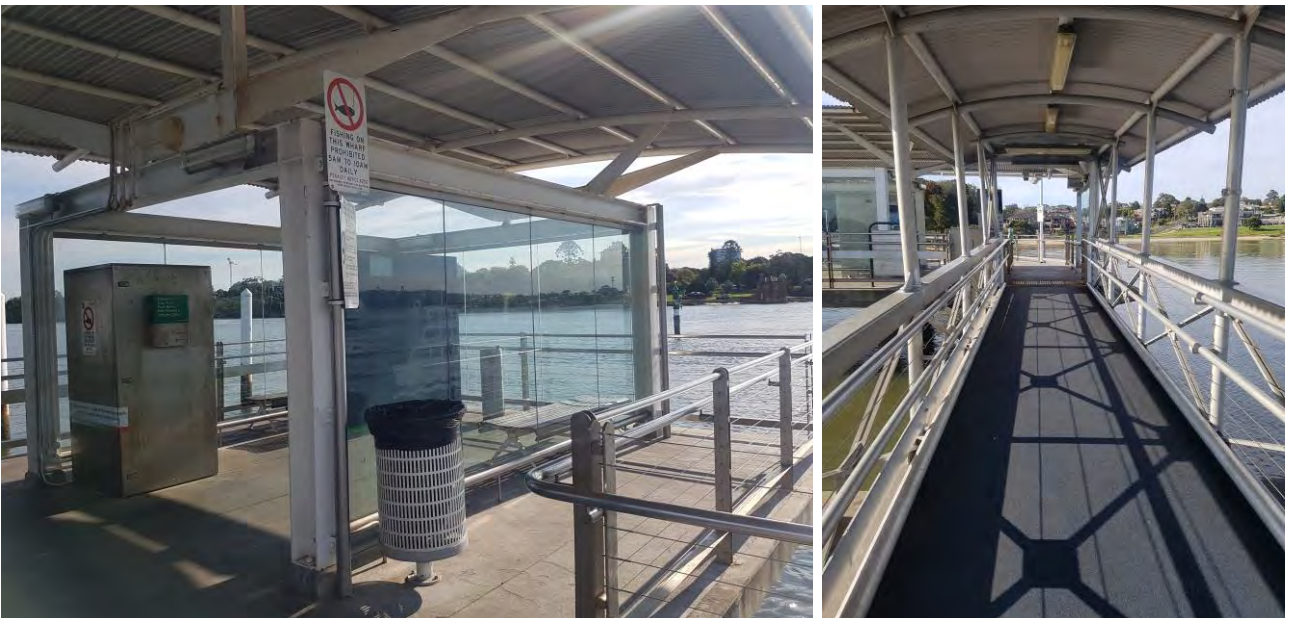
Figure 28: Left – Steel-framed glass panels provide wind protection; Right – A steel-framed gangway connects to a floating pontoon with concrete deck supported by steel piles
