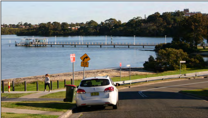
Figure 23. Kissing Point Park (East) with pedestrian/cycle connections in the form of a shared path
