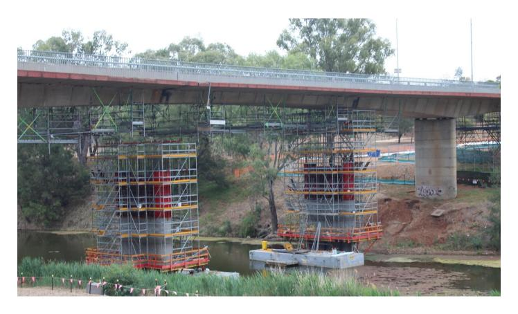
Maintenance work on the LH Ford Bridge commenced in December 2018 and is nearing completion, with the next step in construction to include connecting the new piers to the existing bridge span.
