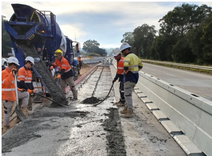
To date, more than 34,000 tonnes of concrete pavement has been placed to build the new lanes on the M1
