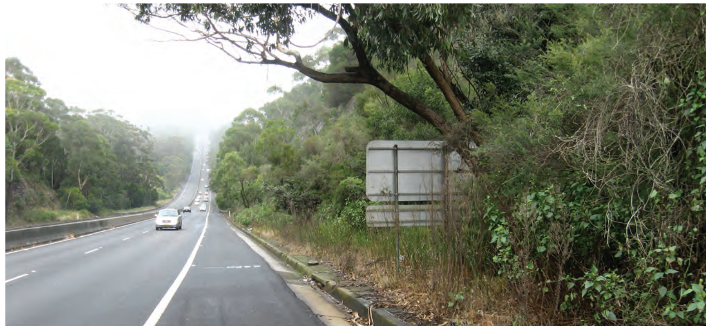
Existing M1 Princes Motorway looking north
