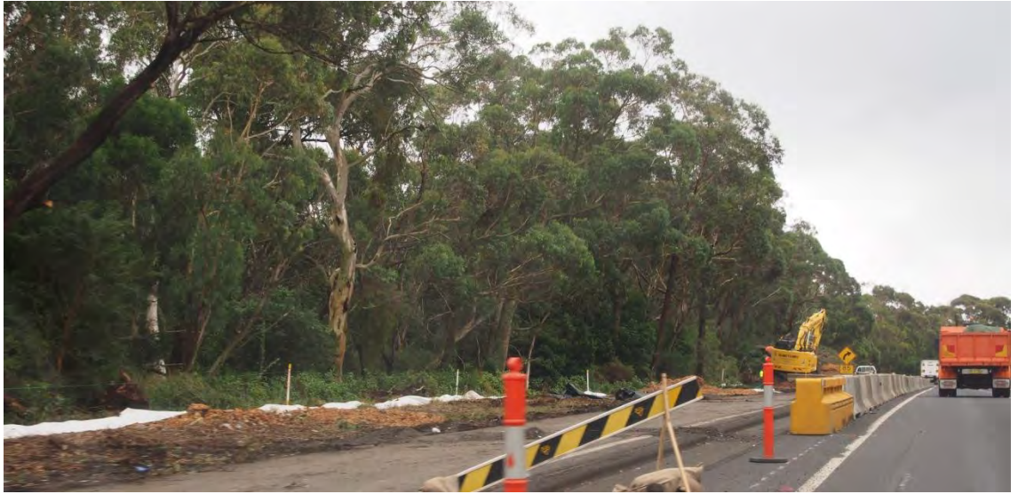
Figure 20 – Picton Road Acceleration works
