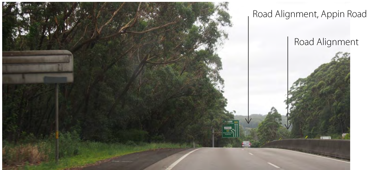
Figure 33 – View to Appin Road
