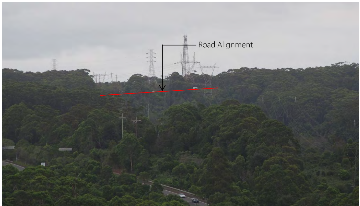
Figure 23 – Zoomed view from Appin Road Overbridge
