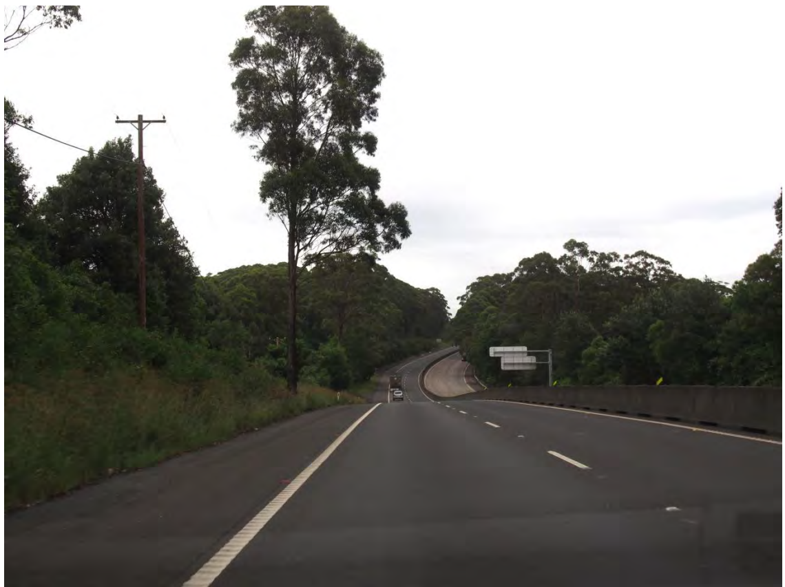
Figure 24 – View point 2 at start of the south bound climbing lanes
