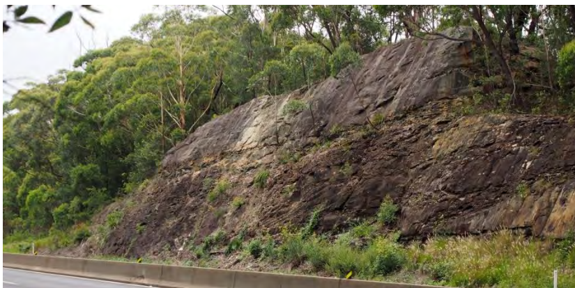
Figure 34 – Existing rock cutting within the alignment
