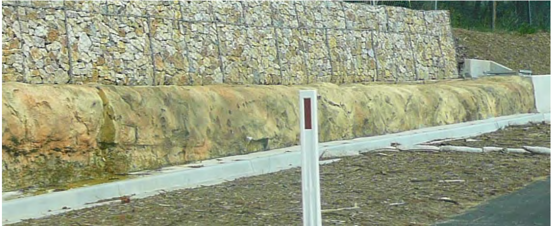
Figure 47 – Faux Rock on leading edge of cutting at Wentworth Falls
