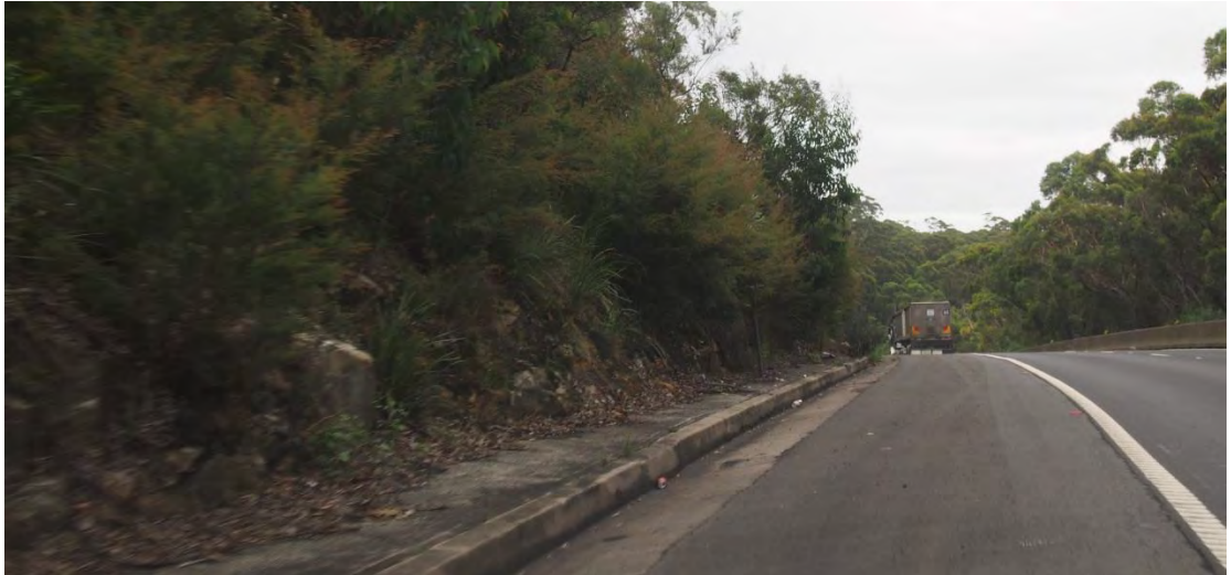
Figure 52 – Verge to base of cutting.
