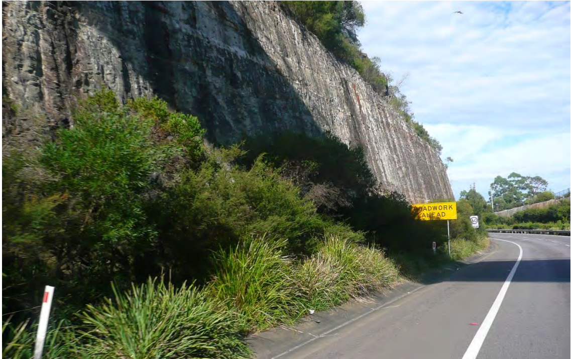
Figure 36 – Existing cutting on Woodford bends with planting to base of cutting
