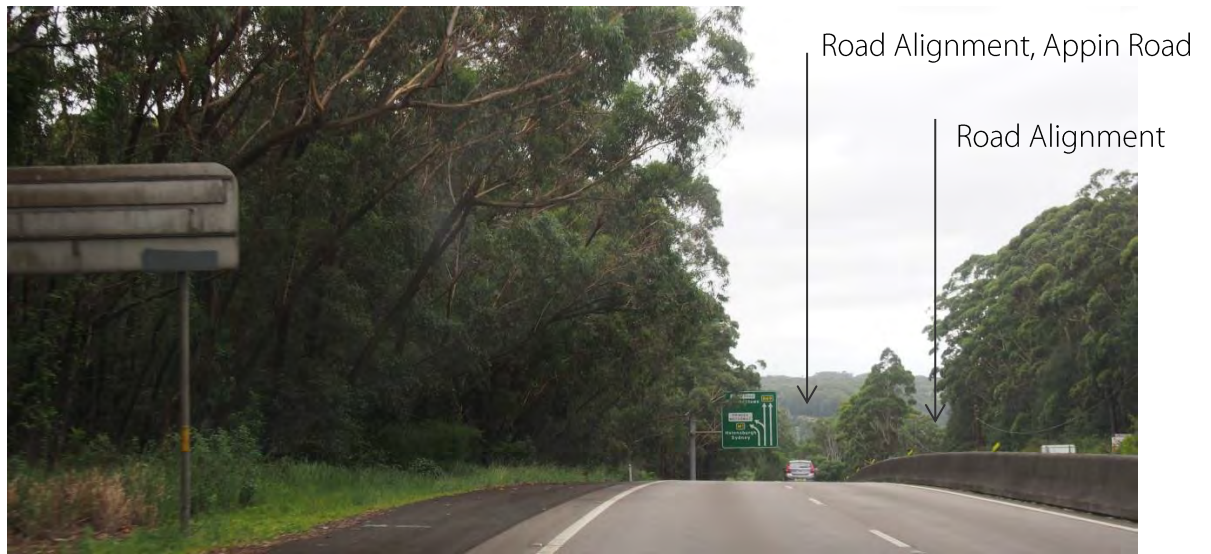
Figure 33 – View to Appin Road
