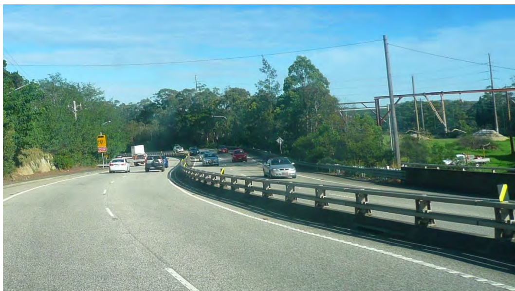
Figure 50 – Double Rail median barrier used on the Woodford Bends, Great Western Highway, The Blue Mountains.
