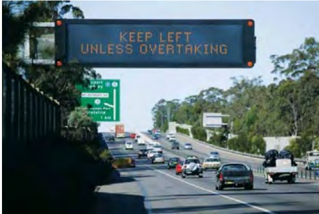
Figure 51 – VMS sign on the M5 Motorway (Source: Roads and Maritime Services)
