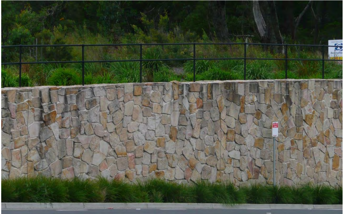
Figure 45 – Stone cladding to pile wall with shotcrete face, Wentworth Falls
