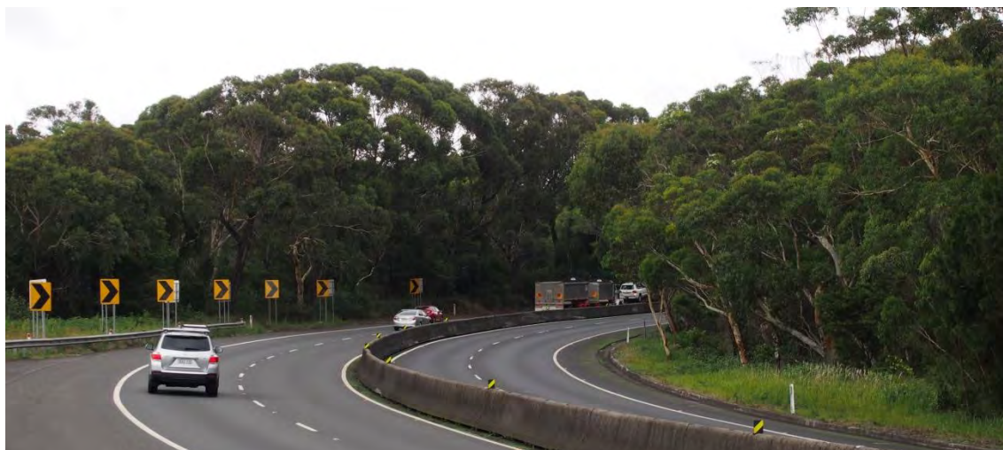
Figure 19 – Zone 3B - Exposed Sandstone Scribbly Gum woodland defines the corridor.
