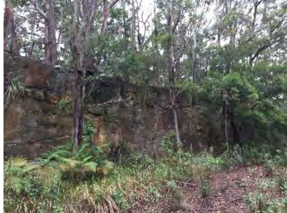
Figure 39: Sandstone cutting near old road alignment, northwest aspect
