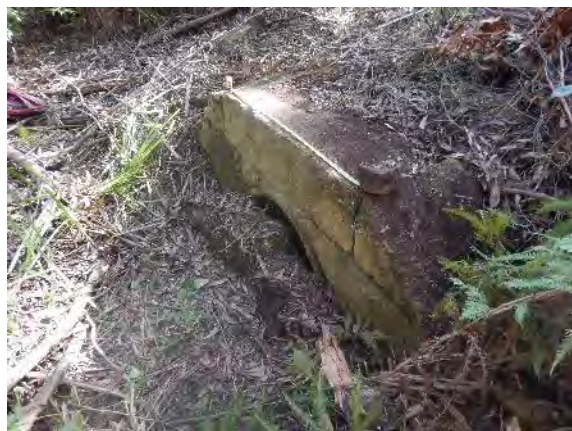
Figure 41: Sandstone culvert, cleared of vegetation, southwest aspect
