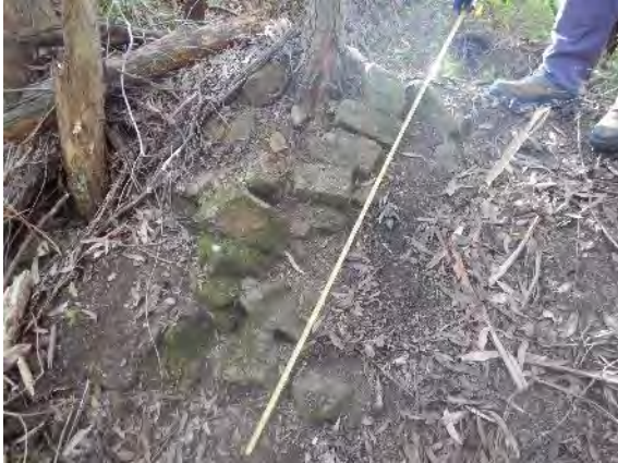
Figure 42: Sandstone retaining wall, west aspect
