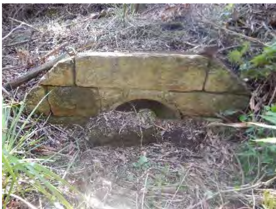
Figure 40: Sandstone culvert, cleared of leaf litter, west aspect
