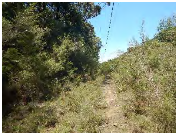
Figure 29: Transmission line in IELA, south aspect
