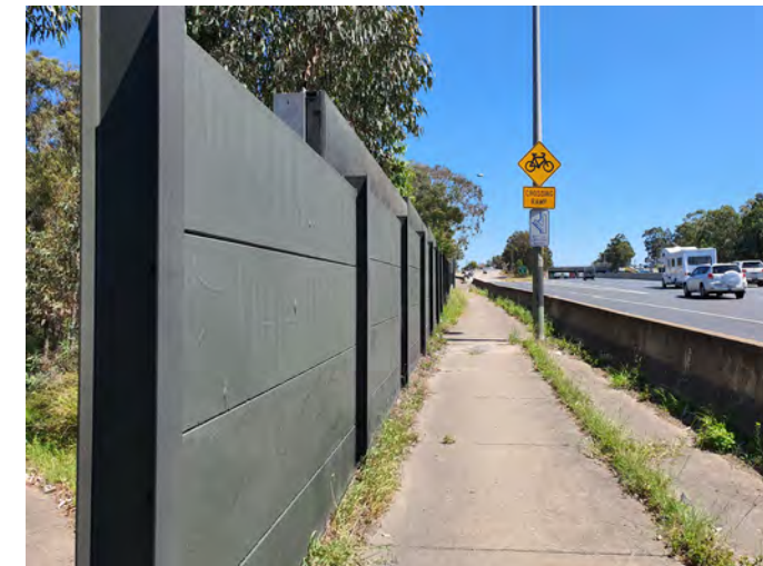
Figure 5.20 The existing noise wall includes older style concrete panels and a new version behind using recycled materials.
