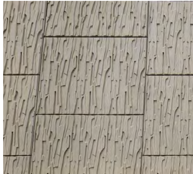
Figure 5.10 Pattern of the precast concrete panels of the existing reinforced earth abutment wall of the existing bridge.
