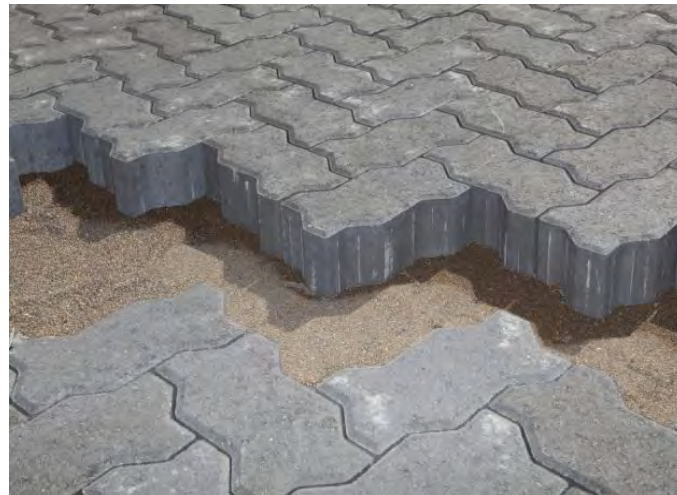
Figure 5.21 Example of interlocking concrete pavers proposed for the spill batters at the abutments.
