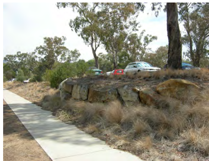
Figure 5.1 Example of drystone boulders ("rock retainers") used to minimise impacts to levels around trees
