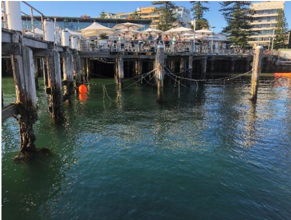
Figure 33: view of the timber piers structure of Wharf 3, looking east (Artefact, 2021)
