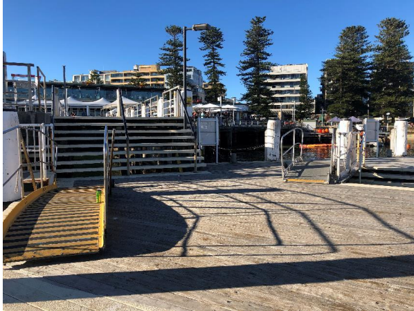
Figure 37 Detail view of Wharf 3 timber decking (Artefact, 2021)
