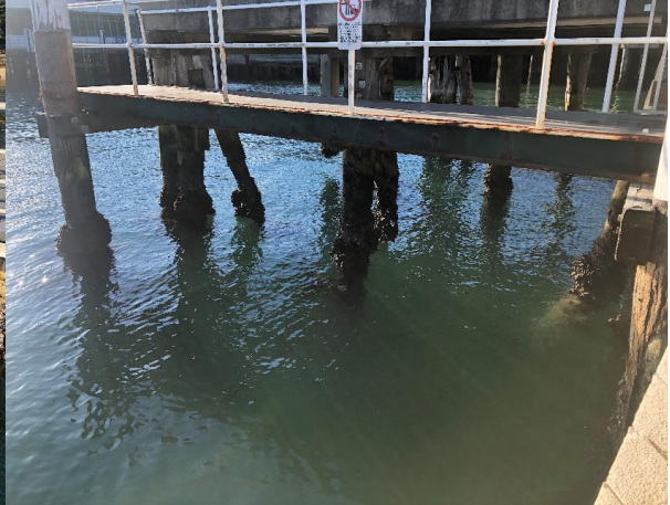
Figure 44 Detail view of gangway from Wharf 3 (Artefact, 2021)
