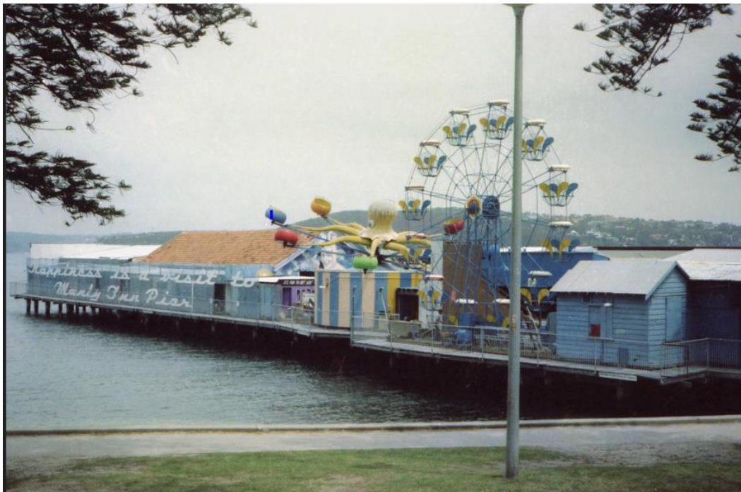
Figure 20: photograph showing Many Fun Pier after the addition of the surrounding walkway added after the Ghost Train fire at Luna Park in 1979, and prior to its demolition in the late 1980's, 22
