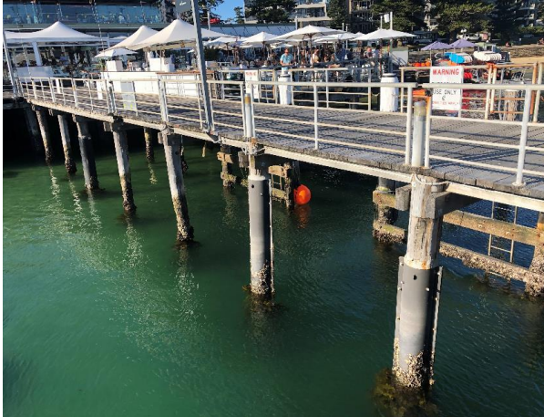
Figure 43 Timber piers on Wharf 3 (Artefact, 2021)
