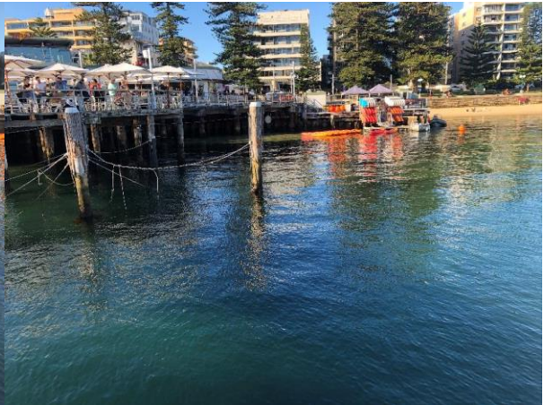
Figure 34: view of the timber piers structure of Wharf 3, looking east (Artefact, 2021)
