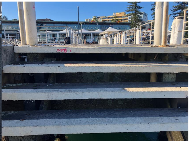
Figure 48 Detail of concrete stairs at Wharf 3 (Artefact, 2021)
