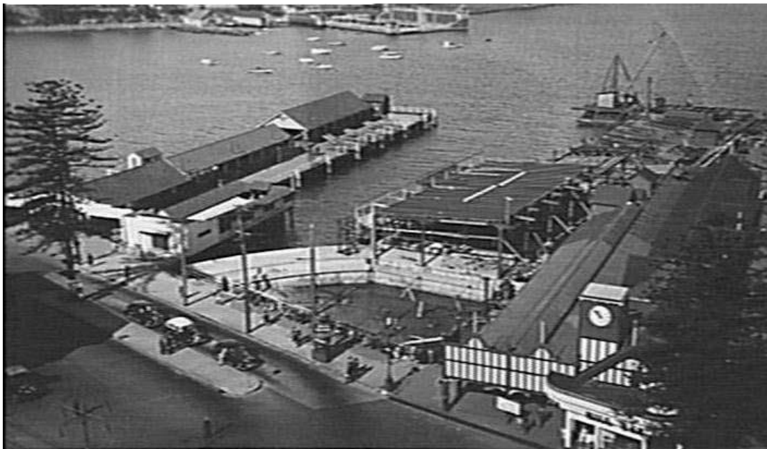
Figure 15: photo of Manly Wharf during construction for the new wharf 1 and 2 dated May 1940. Source: Northern Beaches Council Library Service; courtesy of Manly, Warringah and Pittwater Historical Society.
