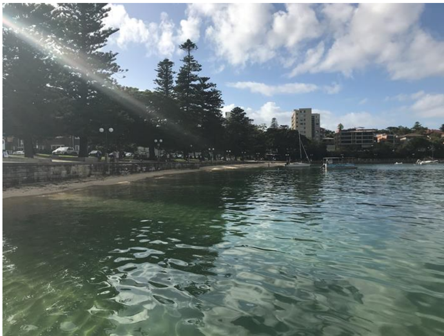
Figure 2-4 Sandflats and vertical seawall near the study area
