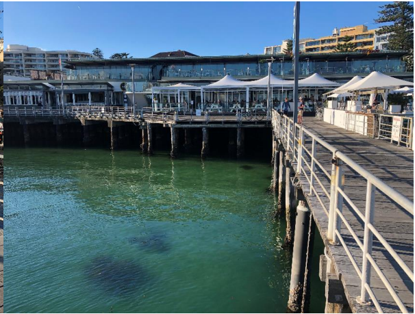
Figure 32: view looking north along the Wharf 3 pier towards the boardwalk and Wharf Bar outdoor seating (Artefact, 2021)
