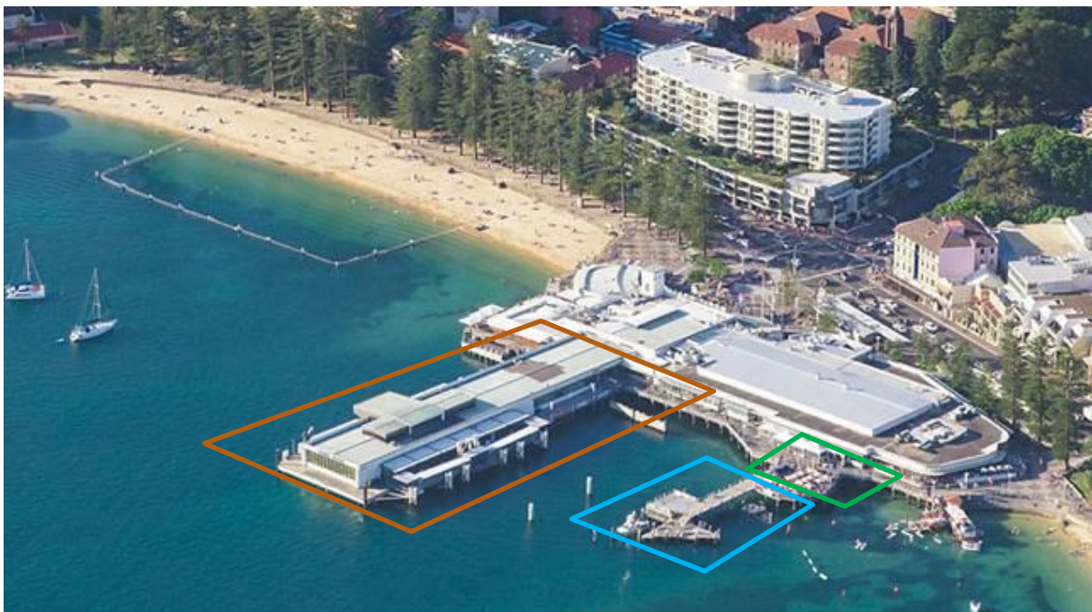
Figure 2: Aerial view of Manly Wharf 1 and 2 (orange), Manly Wharf Bar seating area (green) and Manly Wharf 3 (blue). Source: Northern Beaches Review, 2022 1 with Artefact overlay
