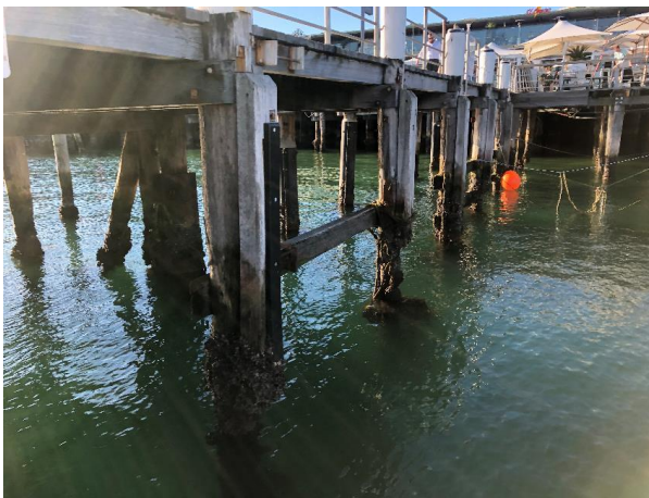
Figure 45 Substructure: Wharf 3 (Artefact, 2021)
