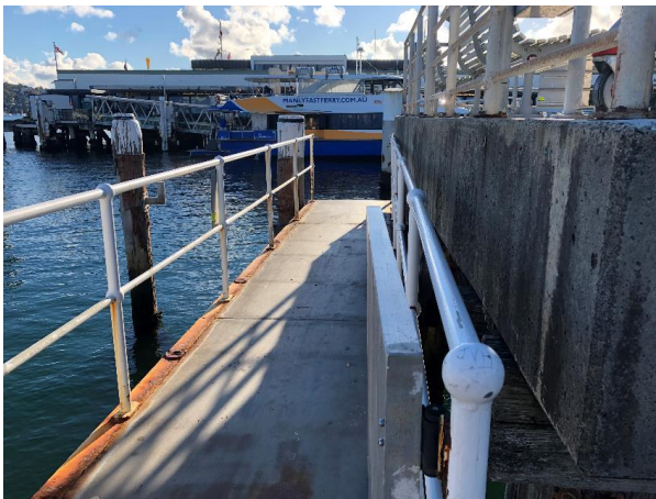
Figure 47 Concrete ramp down to Wharf 3 (Artefact, 2021)
