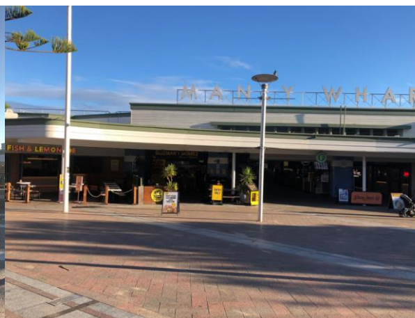
Figure 30: Entrance to Manly Wharf from Belgrave St / East Esplanade. Photograph taken looking southwest (Artefact, 2021)
