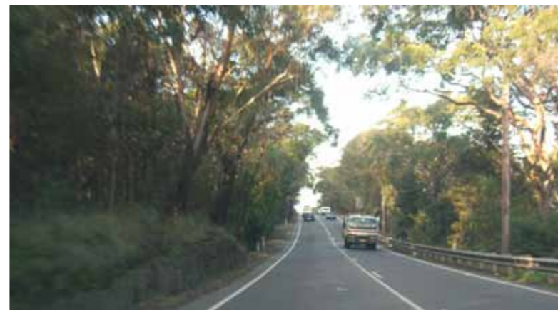
View east, constrained section at the top of the ridge with steep drop off to Garigal National Park on the right.
