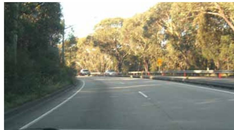
Curving left hand drive up around the Baha'i Temple site, with slow vehicle lane and elsholz kerb.
