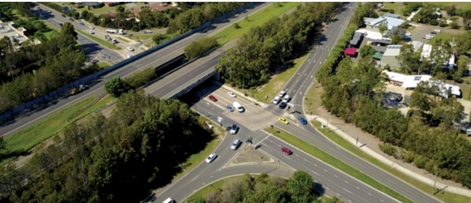
Aerial view of Mulgoa Road and M4 Motorway intersection.
