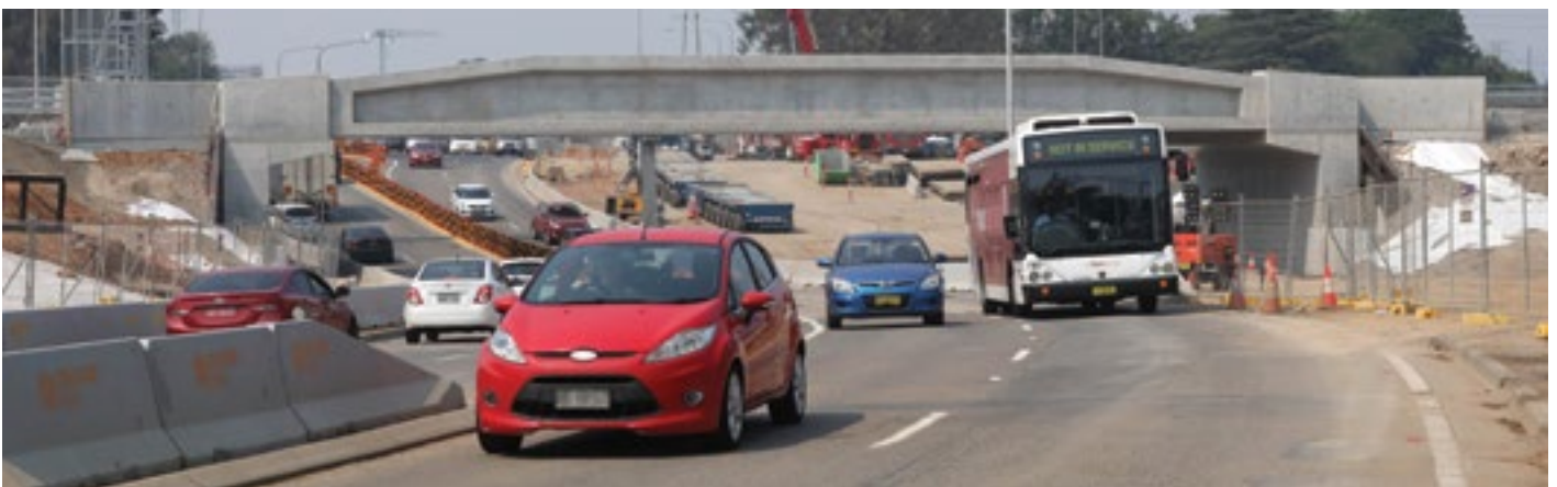
New rail bridge placed over Castlereagh Road
