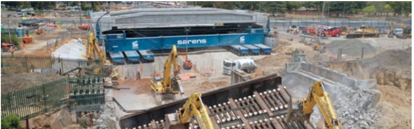
Demolition of existing rail bridge
