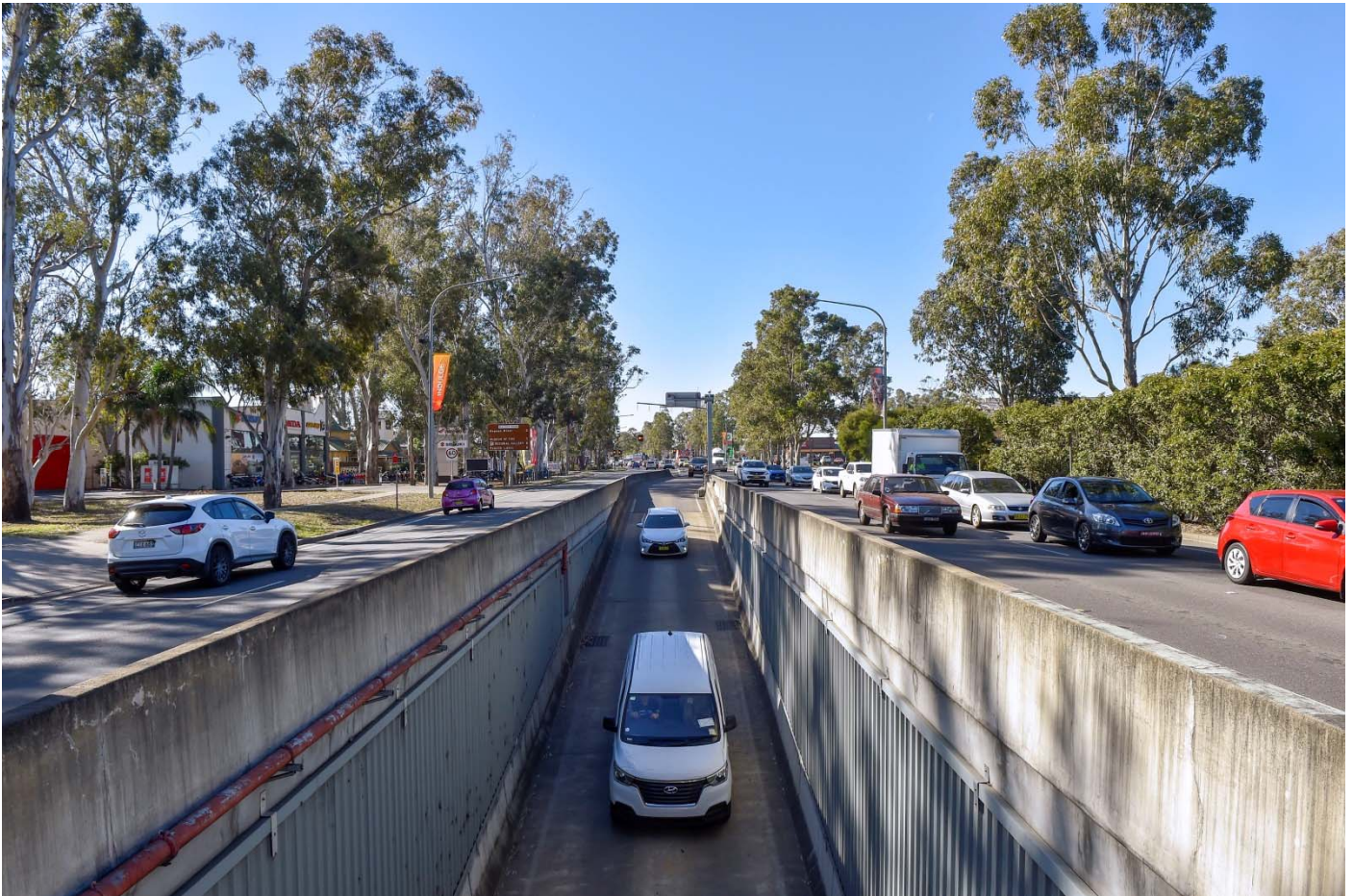
Image of Wolseley Street tunnel on Mulgoa Road, Jamisontown
