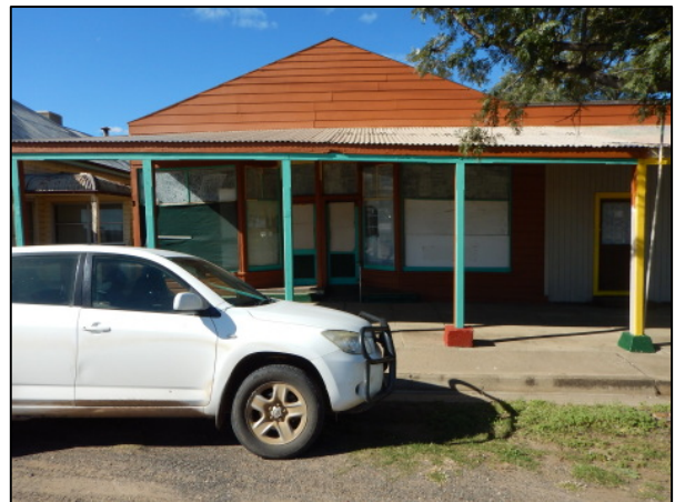
2. Overview of Oldhams Smallgoods building, facing east.
