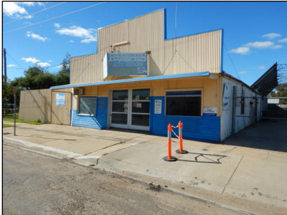
1. Overview of the LS Rowe Stock and Station Agents building, facing northeast.
