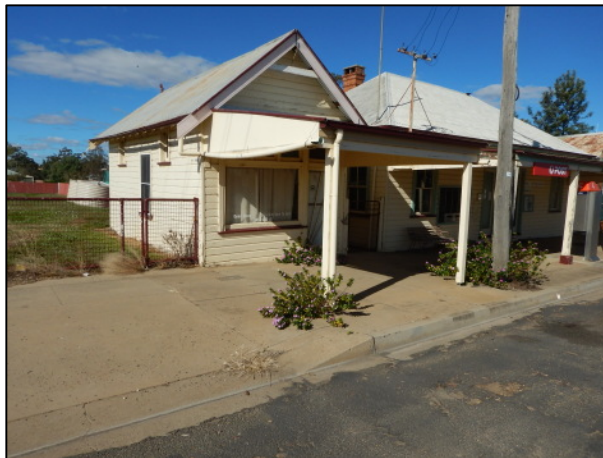
1. Overview of AB Meppem & Co building, showing the frontage, facing southeast.
