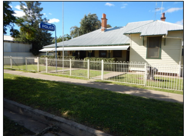
2. Overview of the Bellata Police Station building, facing east.
