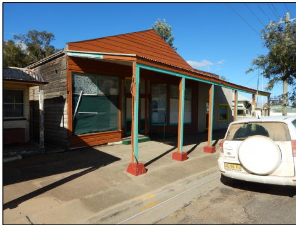
1. Overview of Oldhams Smallgoods building, facing southeast.
