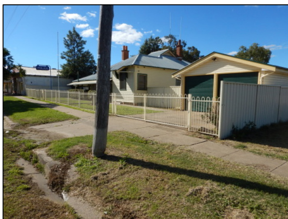
3. Overview of the Bellata Police Station building, facing northeast.
