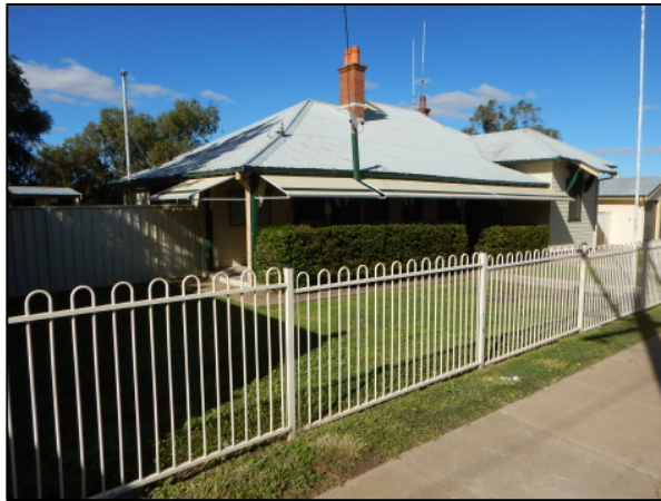
1. Overview of the Bellata Police Station building, facing southeast.
