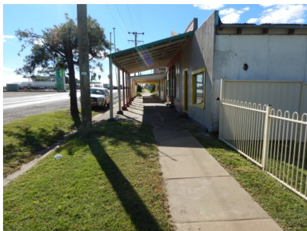
4. Overview of Oldhams Smallgoods building, facing north.
