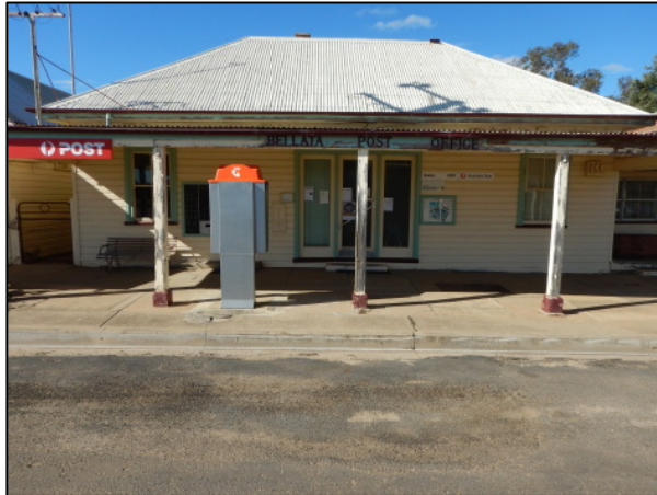
1. Overview of the Bellata Post Office building showing the building frontage, facing east.
