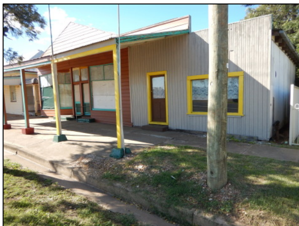
3. Overview of Oldhams Smallgoods building, facing northeast.
