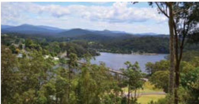
View of the current bridge from the east
