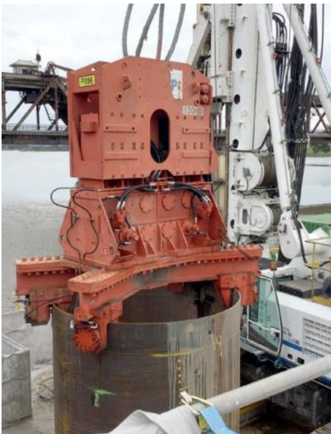
Example of a piling hammer vibrating a steel casing into place
