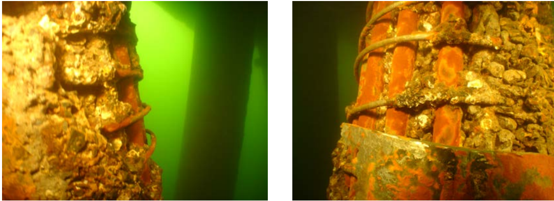
Figure 2. Underwater inspection of Nelligen Bridge Piers
