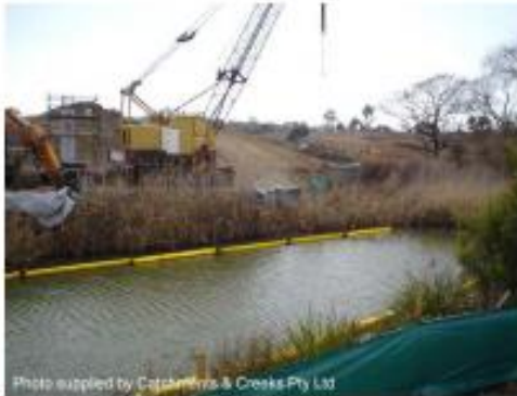
Photo 1 – Silt curtain used as an isolation barrier
