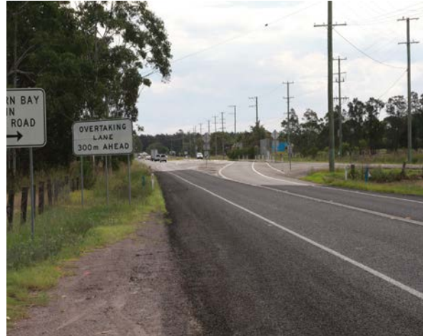
View west to tie-ins with dual carriageways near Cromarty Lane
