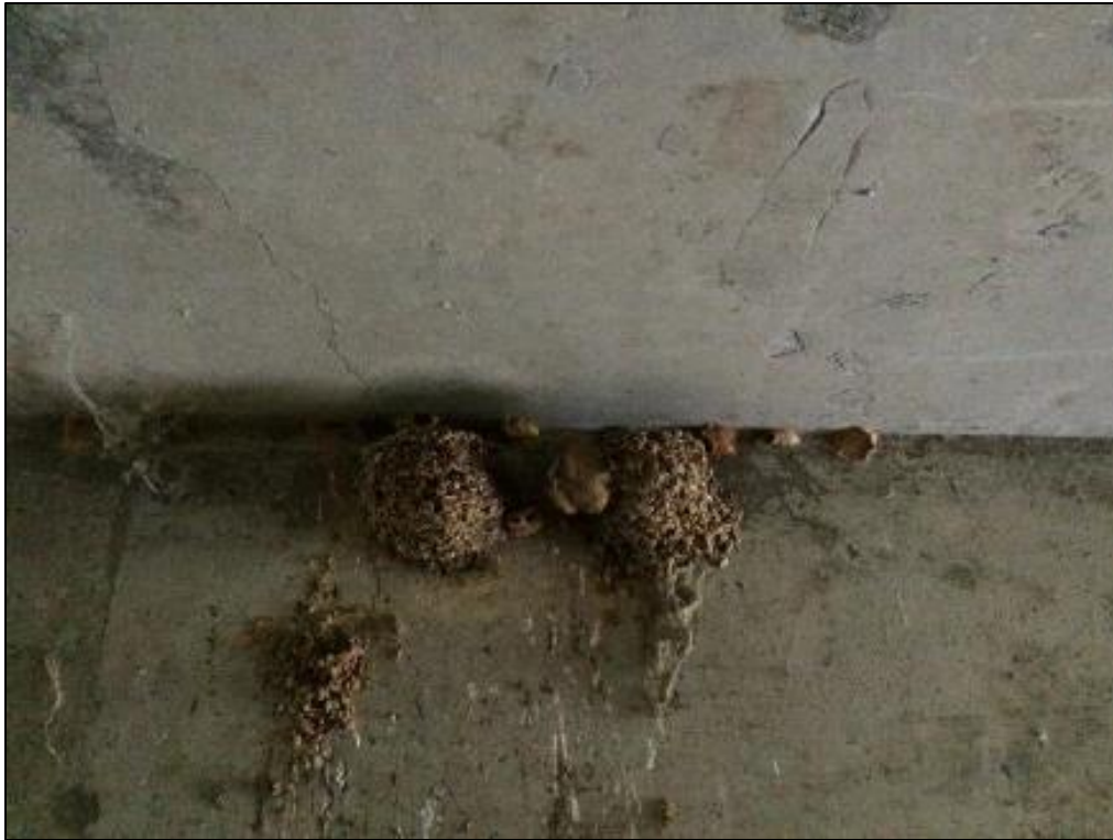
Plate 10: Box Culvert with Swallow's Nest
